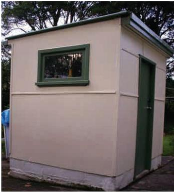
Figure 1: Bonded Asbestos (Fibro)
