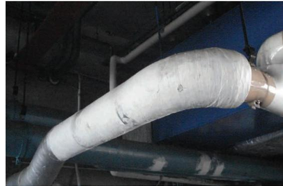
Figure 3: Friable Asbestos – Pipe Lagging
