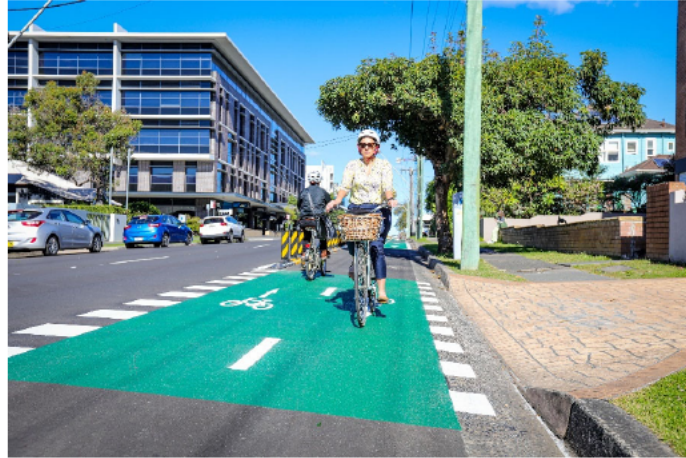
[IMAGE: Dedicated cycleway as part of the Pop-Up Cycleways project, Kembla Street, Wollongong
