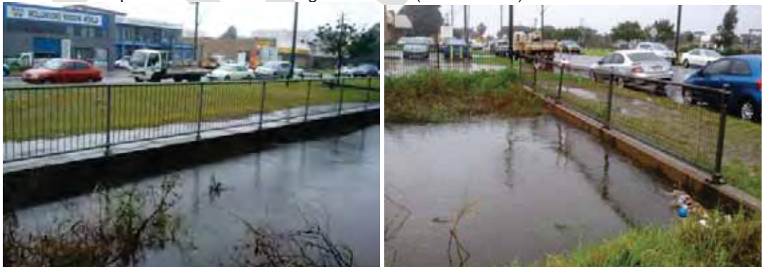
Photo 4: Example of backwater flooding at a culvert (Swan Street)
