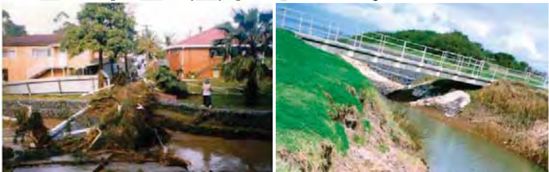
Photo 1: Small bridges affected by varying levels of debris blockage
