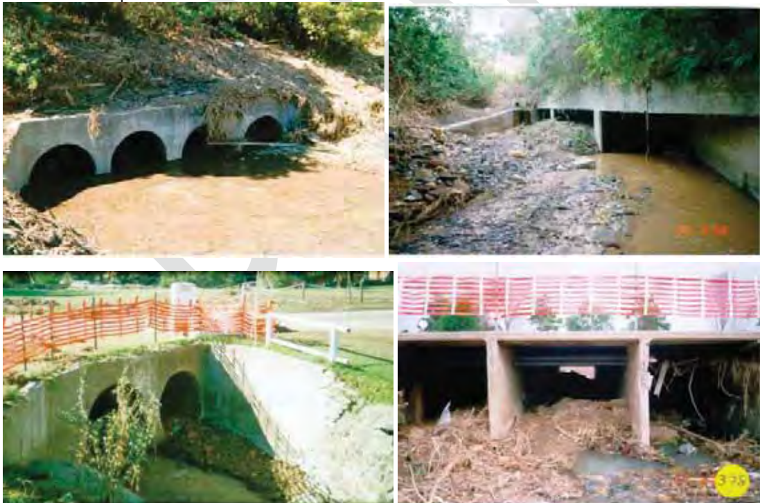
Photo 3: Examples of sedimentation within culverts
