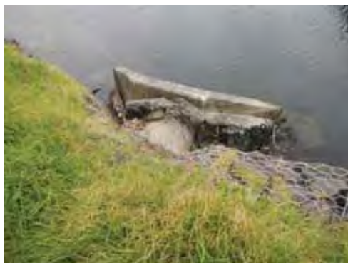
Plate 14 Stormwater pipe headwall
