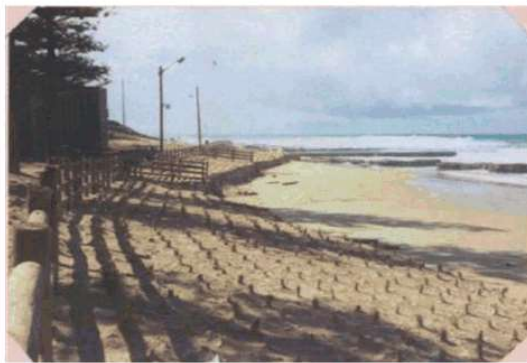
Photograph 4: Dune stabilisation work in 1986 (GHD, 2014 courtesy of Ian Foreman).
