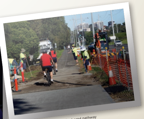
Construction of Puckey's shared pathway
