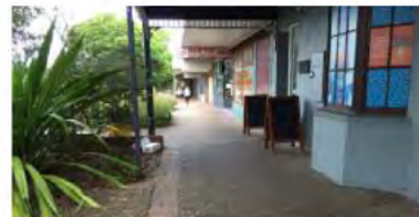
Poor interface public space and adjacent shops
