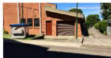
Pedestrian access between Club Lane and Walker St, adjacent to the community centre
