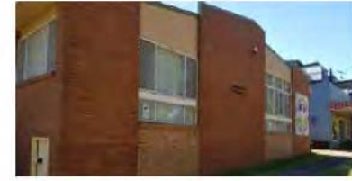
An addition at the front of the community centre does not address Walker Street
