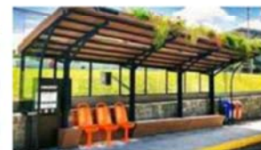
UPGRADED BUS SHELTER
