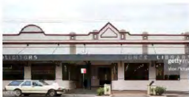
Example of an historic shopfront presented to the street: Junee Library
