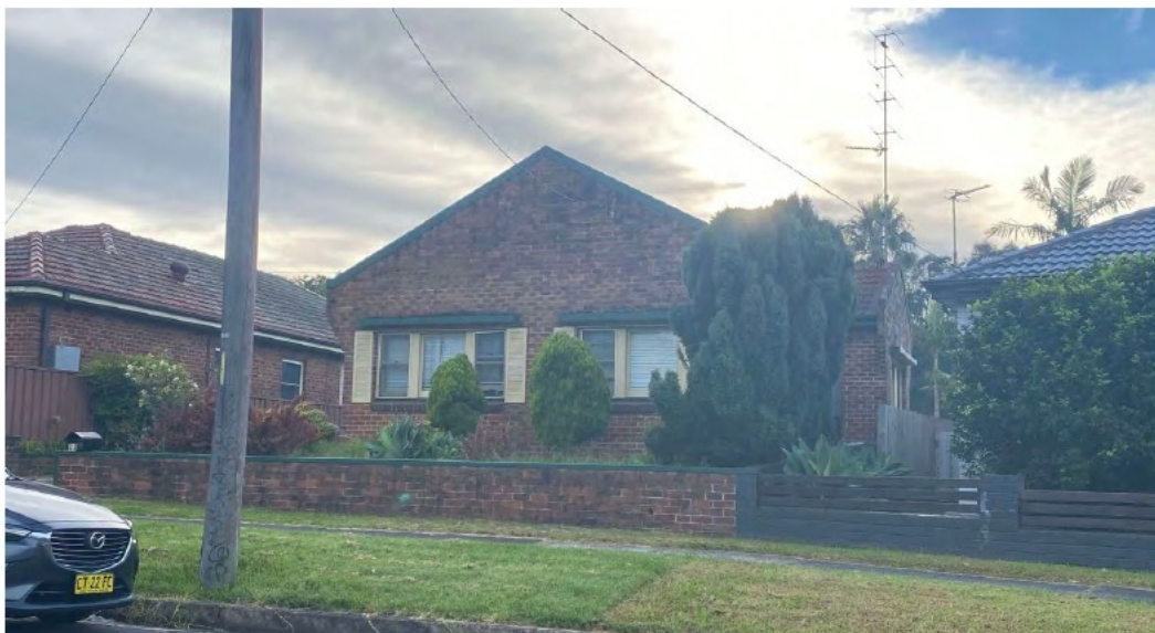
Figure 20 – Dwelling of similar materiality and built form at 23 Crawford Avenue
