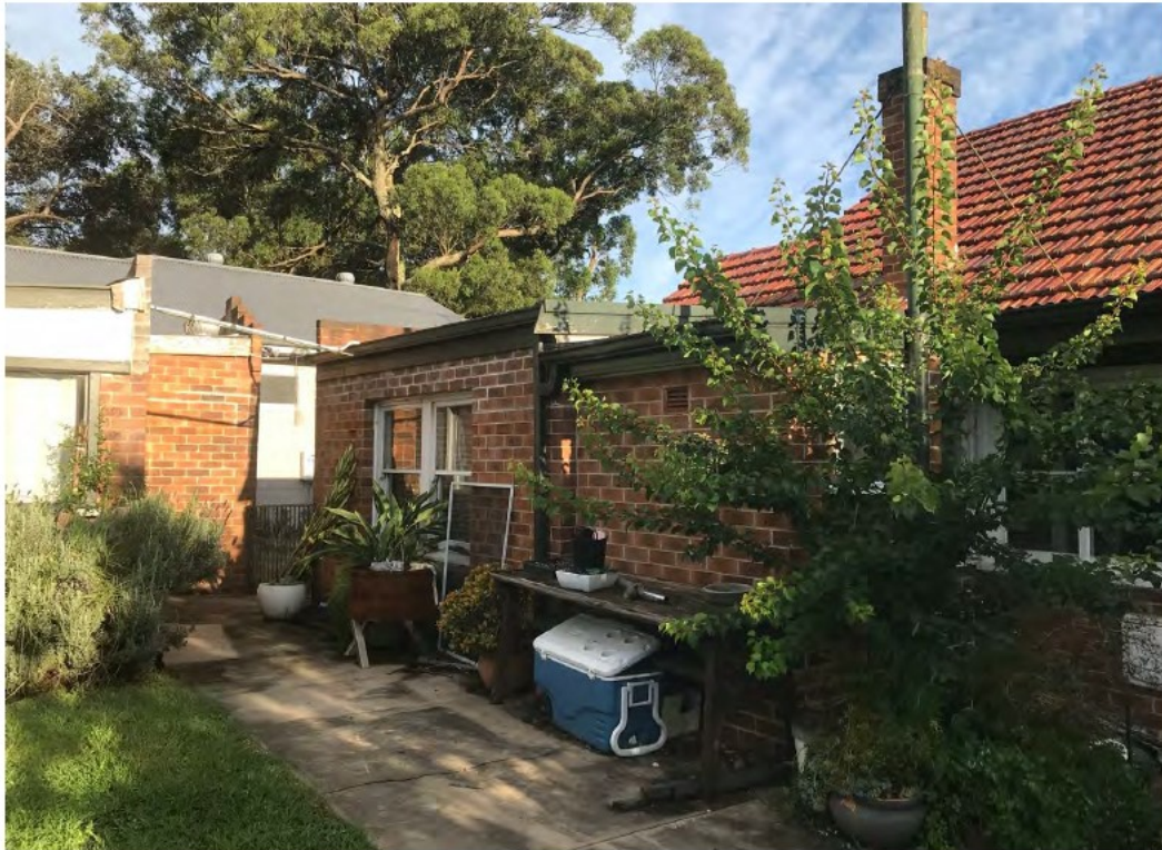
Figure 11 – More recent extension to main dwelling (Corona Projects, 2021)
