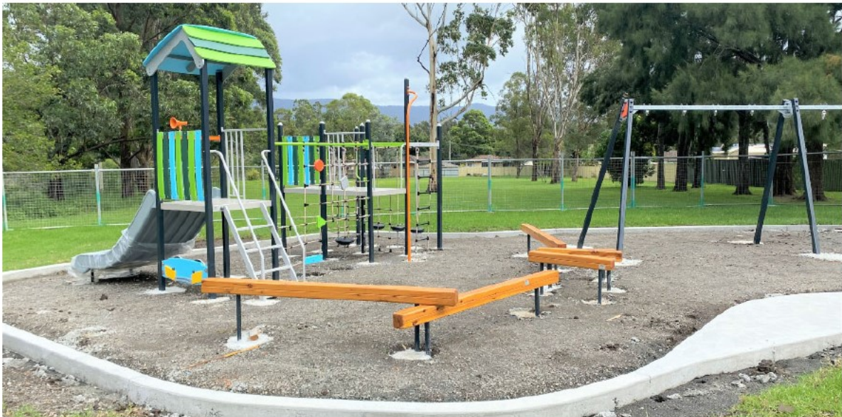
[IMAGE: Playground works in progress at Cormack Street Reserve, Dapto]
