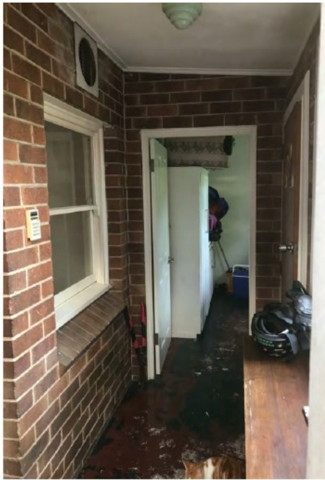
Figure 16 – Non-original rear extension (Corona Projects, 2021)
