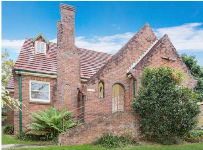
Figure 5.4 342-344 Lawrence Hargrave Drive, Thirroul
