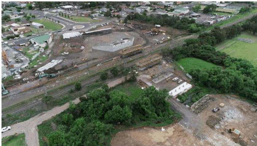
[IMAGE: A significant milestone in the Fowlers Road to Fairwater Drive road link will be reached in January when the pre-cast concrete 'Super T' girders are placed over the section of the bridge spanning the South Coast rail line.]
