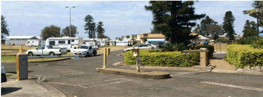
Entry area and boom-gates
