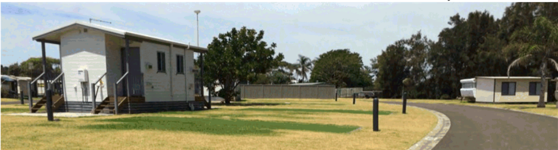
BELOW En-suite facilities and sites
