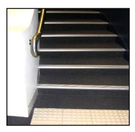
Figure 13: Correct enclosed opaque risers with no overhangs which meet the requirements of stairways suitable for people with disabilities, under AS1428.1.
