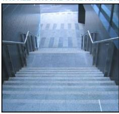
Figure 18: The correct interpretation of the requirements for TGSIs on an intermediate landing with no handrail break: there are no TGSIs on the landing.
