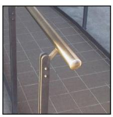
Figure 5: (Top left) Handrails which do not comply with the specifications of AS1428.1 for handrails on stairs suitable for people with disability since the handrails fail to return to a side wall or downwards and back on themselves at 180°.
