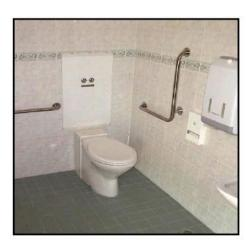
Figure 30: The incorrect placement of the toilet paper holder too far forward of the WC pan, which forces patrons to lean excessively forward to get to the paper. This can result in patrons falling off the pan in attempting to reach the toilet holder.
