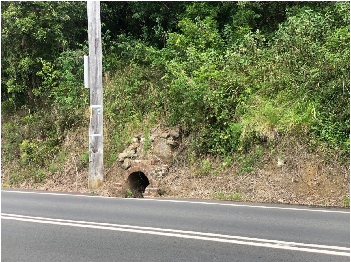
Photo 5 – Looking west across LHD to drainage outlet
