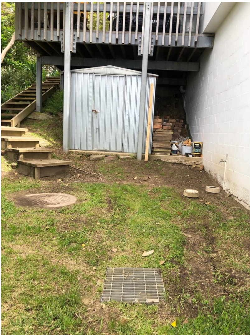
Photo 8 – Underside of existing carport (to be developed)
