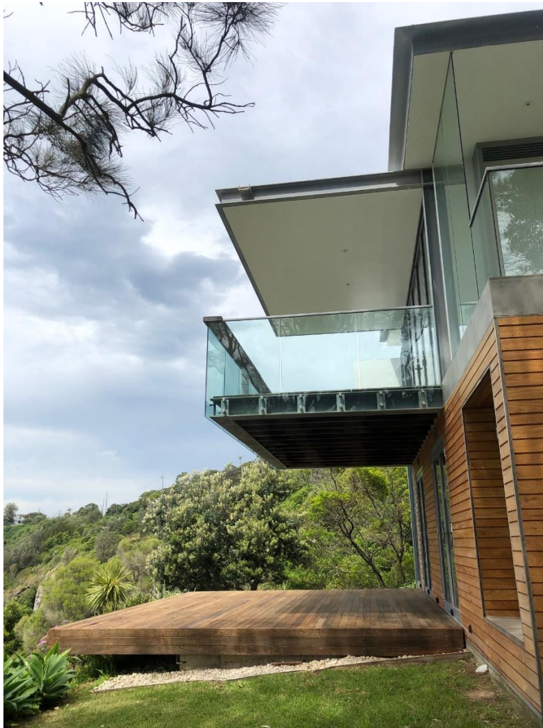
Photo 15 – Looking south (from rear of No 347 LHD)
