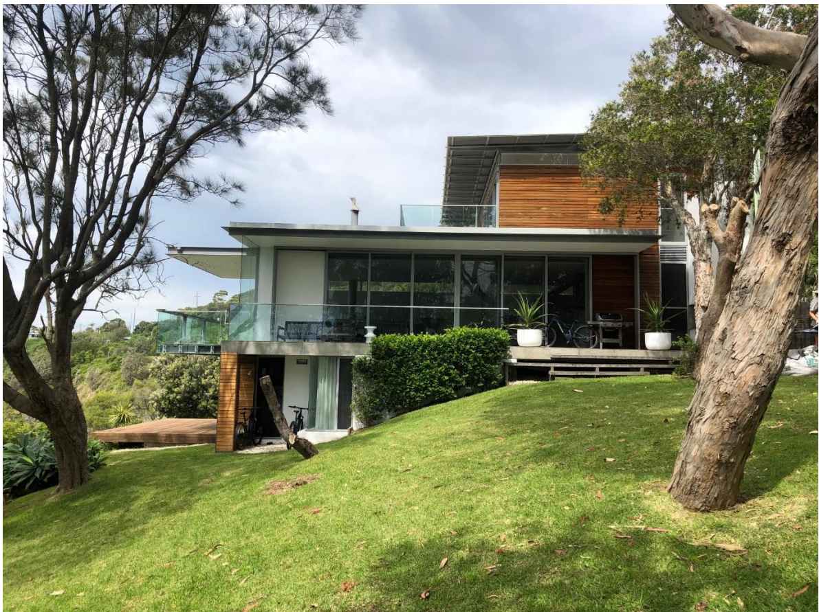
Photo 14 – Looking south (from RE1 block) and towards No 347 LHD (north elevation)
