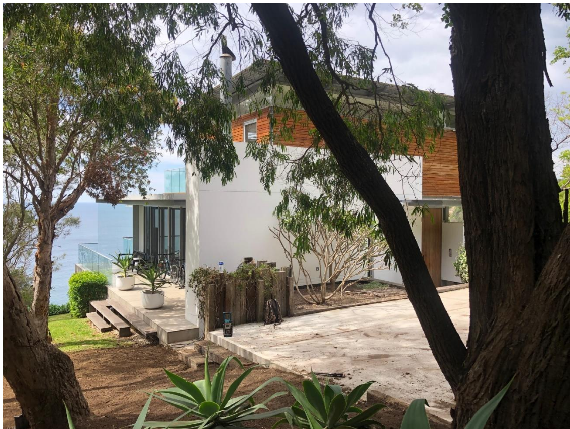
Photo 15 – Looking east (from RE1 block) and towards NW corner of No 347 LHD
