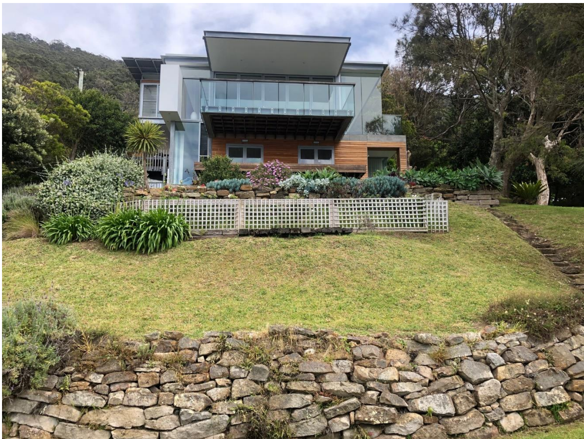
Photo 19 – View to east elevation of No 347 LHD
