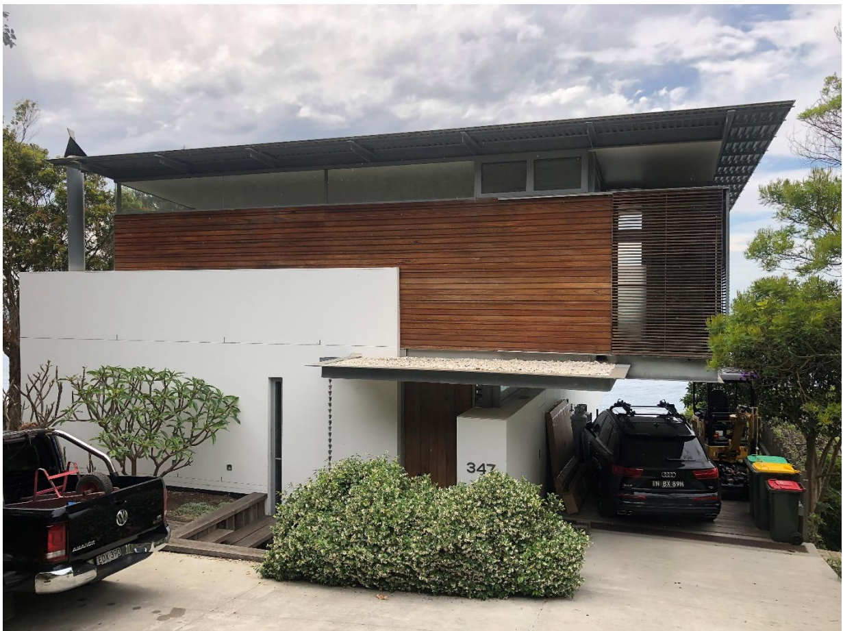
Photo 2 – West elevation existing dwelling (facing LHD)
