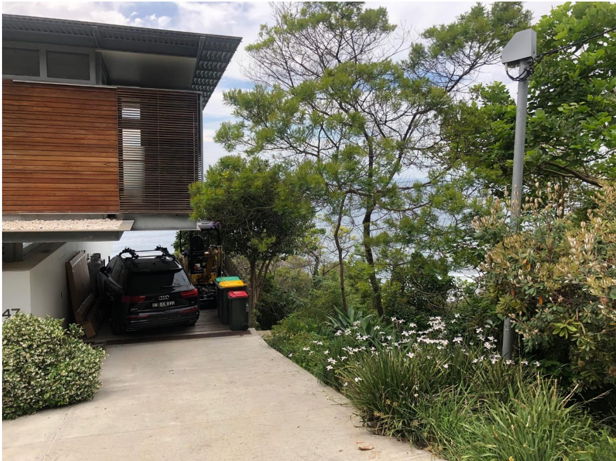
Photo 7 – View from driveway looking east (driveway area to be developed & 4 trees removed)
