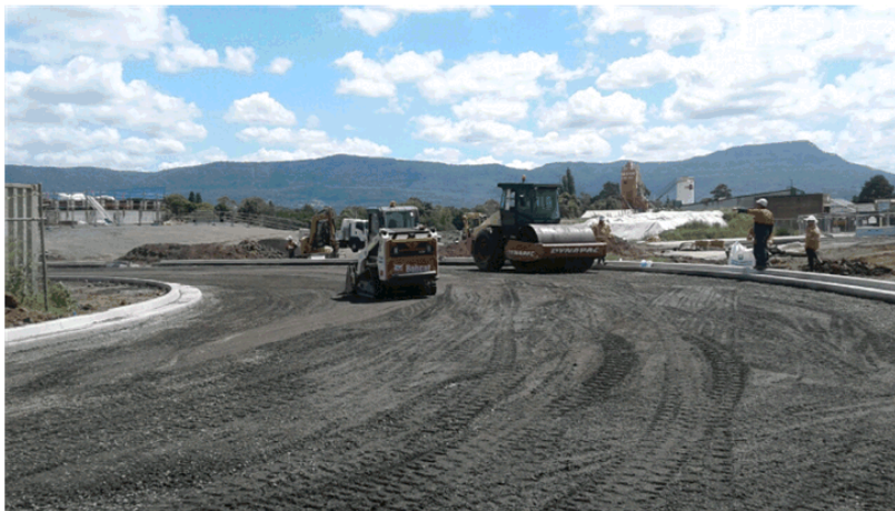
[IMAGE: Works on the Marshall Street deviation project, West Dapto]
