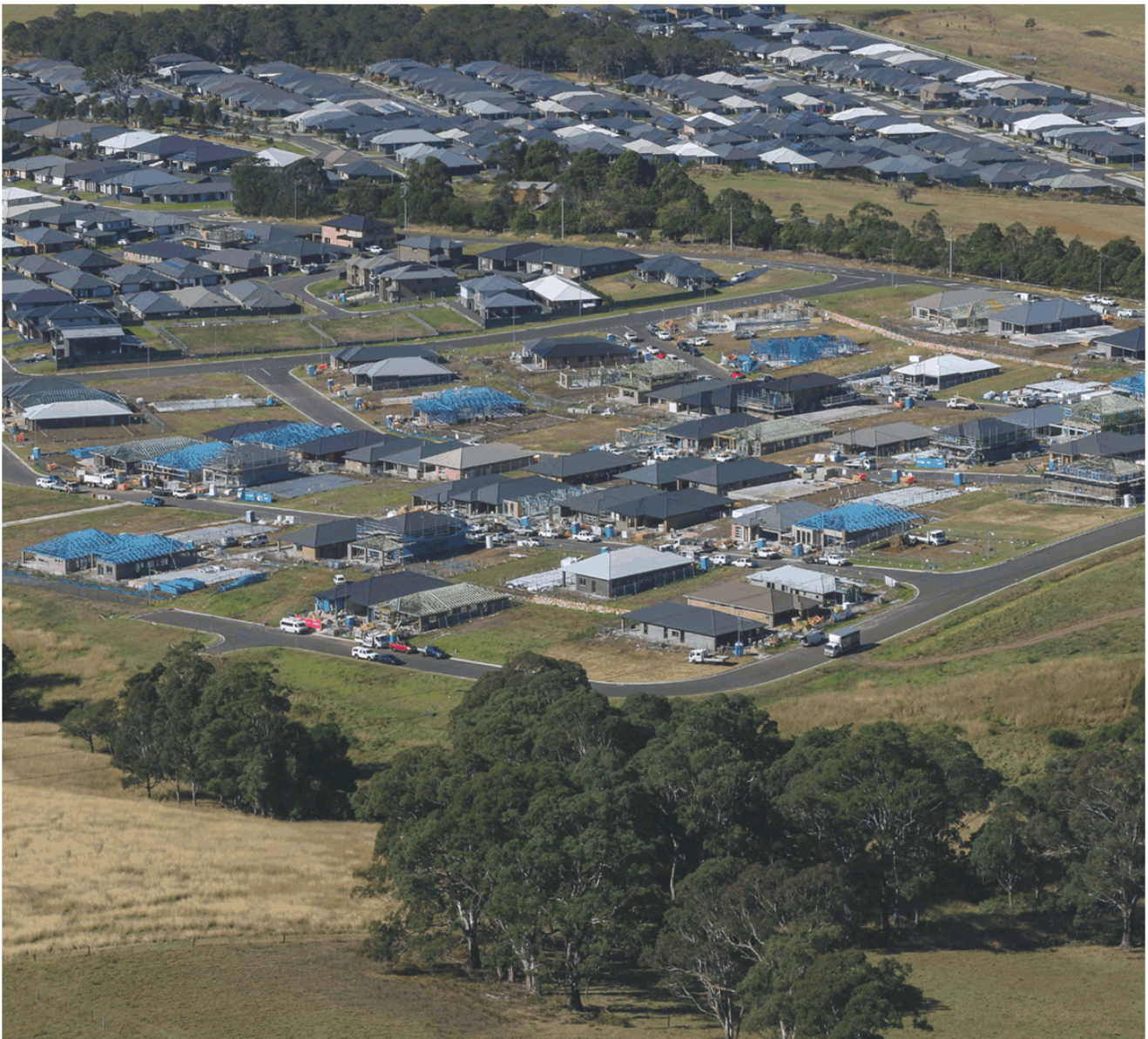
Housing development in Horsley.
