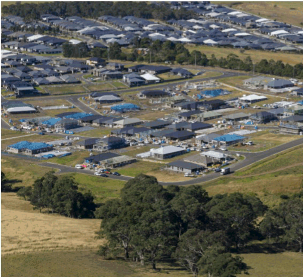
Housing development in Horsley.
