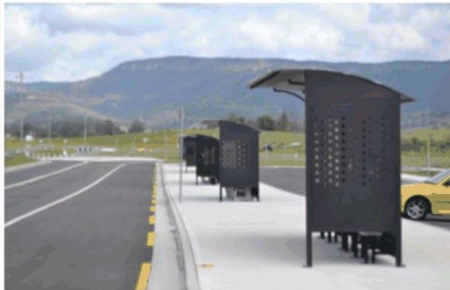
Dapto High School Bus Interchange ($2.4 million). Bus stops and drop-off areas, increasing access and safety.
