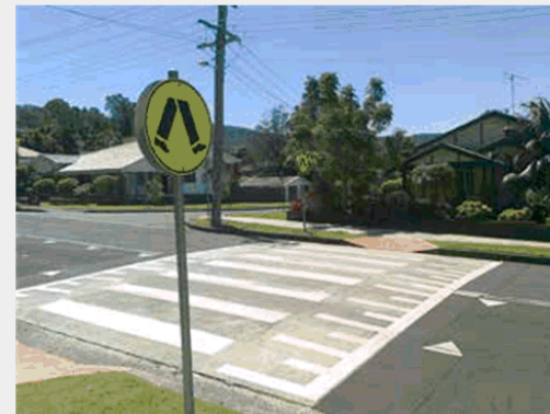
Marked foot crossing on raised platform
