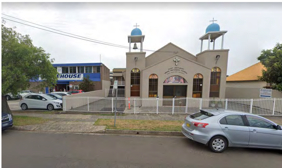
Figure 3: Site photo showing adjacent church with 5.5m setback to its northern boundary
