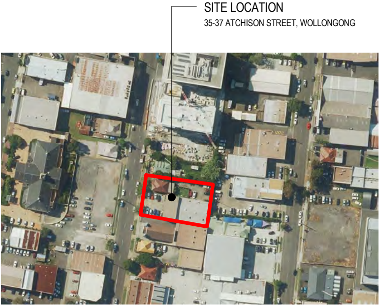
AERIAL PHOTOGRAPH 35-37 ATCHISON STREET, WOLLONGONG
