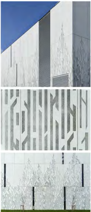
EXAMPLE IMAGES OF GRAPHIC CONCRETE TREATMENT
