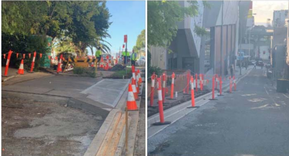
[Image: New footpath completed along Crown Lane and Regent Street, Wollongong]
