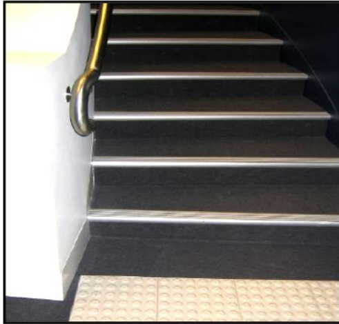
Figure 13: Correct enclosed opaque risers with no overhangs which meet the requirements of stairways suitable for people with disabilities, under AS1428.1.
