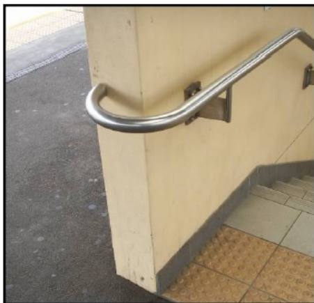
Figure 7: (Top left) Correct return of the handrail to a side wall and the required 270° top arc clearance.
