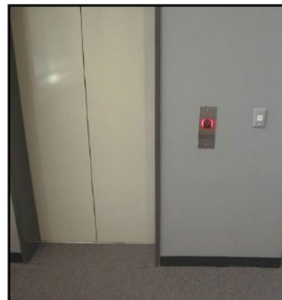
Figure 20: (Top left) Show call buttons which comply with the requirements of AS1735.12 in terms of their placement, luminance contrast application and raised tactile and Braille which are consistently placed adjacent to each button.
