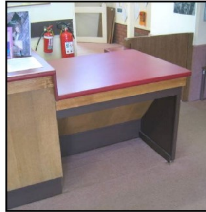
Figure 26: (Top left) Reception counters which allow for a frontal approach with an adequate toe plate and knee space for a person using a wheelchair.
