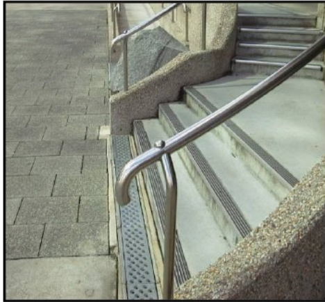
Figure 5: (Top left) Handrails which do not comply with the specifications of AS1428.1 for handrails on stairs suitable for people with disability since the handrails fail to return to a side wall or downwards and back on themselves at 180°.
