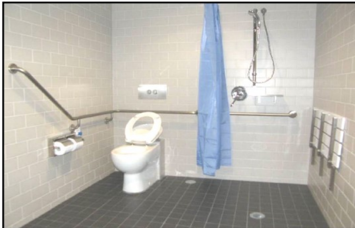
Figure 28: Correct placement of toilet and shower fittings as per the requirements of AS1428.1. Note: The toilet roll holders are placed below the grab rail, to ensure a person using a wheelchair is able to rise off the pan and transfer back onto their wheelchair unencumbered.
