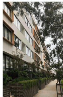
Built environment incorporating greening on public and private land
