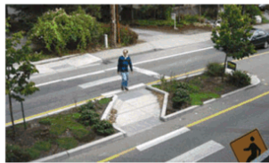
Clearly defined pedestrian bays allow for safe designated crossing points along wider roads.
