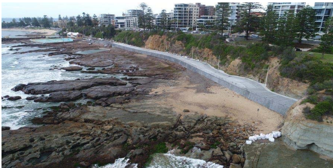
IMAGE: Blue Mile Tramway Seawall path beginning to take shape, March 2018
