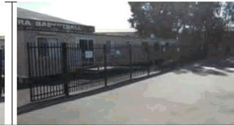
12. Illawarra Basketball Stadium C
