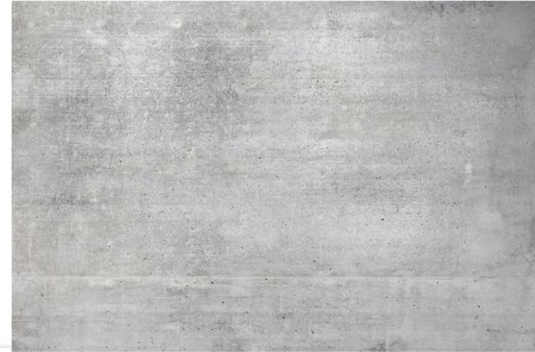
CT-01 OFF FORM CONCRETE
