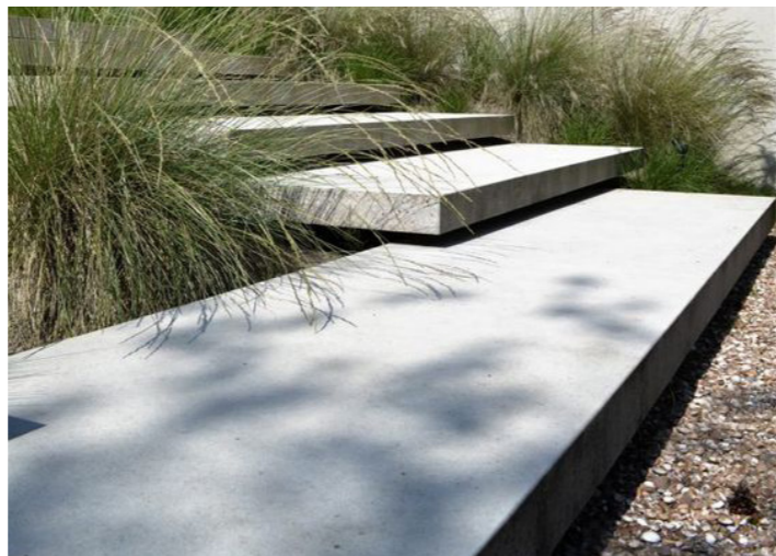
'FLOATING CONCRETE STEPS'
