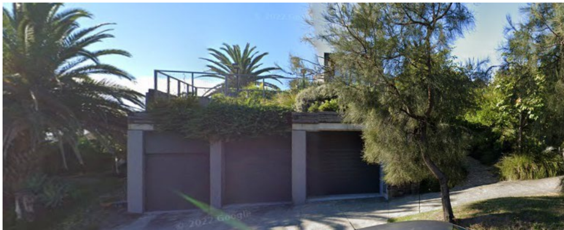
No. 131 Lawrence Hargrave Drive – 2 properties south of subject site. Approx. 3m high garage structure with landscaping and fencing above. No passive surveillance of LHD from dwelling.
