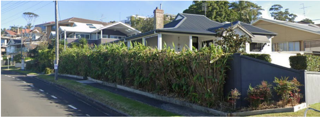
Cnr Oceana Pde & Lawrence Hargrave Drive – western side of LHD. Solid 1.8m fencing with bamboo screen in front, with no passive surveillance of LHD.
