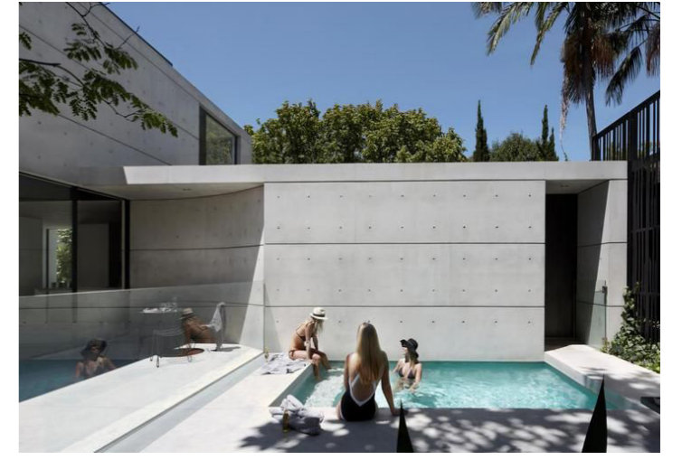
W1 - OFF FORM CONCRETE WALL
