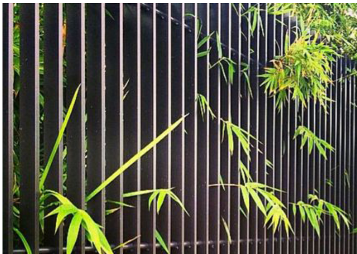
F4- 1.8m STEEL PALISADE BOUNDARY FENCE
