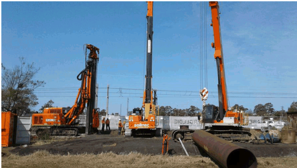
Piling for Bridge 2 work has commenced on the Fowlers Road to Fairwater Drive project.
