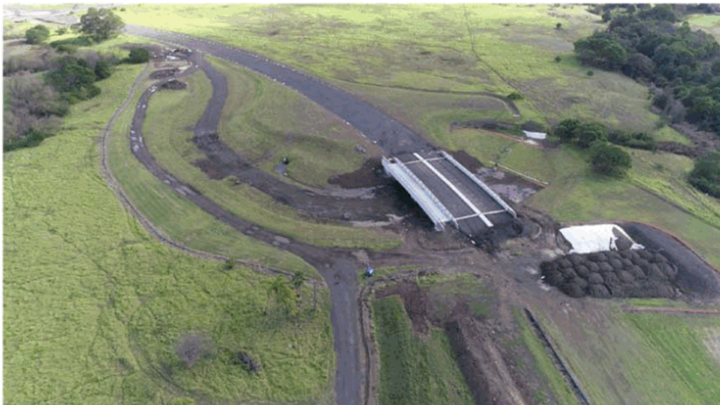
Completed bridge over the flood cut channel at West Dapto – Stage 1E Urban Release area.
