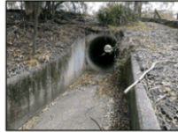
6 ROBSONS ROAD DRAINAGE WORKS Upgrade Robsons Road culvert drainage to reduce flooding impacts to the road and the western part of campus whilst ensuring no greater impacts downstream of the culvert.
