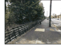
4 RETAINING WALL REPLACEMENT Replace existing timber retainers with quality masonry retaining wall along northside of Northfields Avenue at eastern end.
