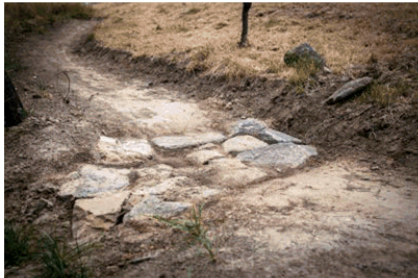
Example – Paved drainage culvert
