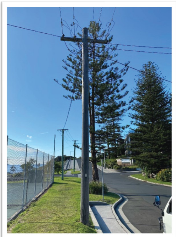
Pole location – Next to Headlands Park
