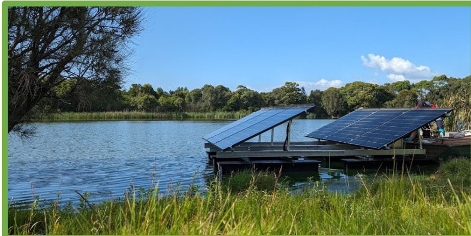
Two solar-powered aeration pumps were installed at Coomaditchie Lagoon to combat a persistent blue-green algal bloom affecting the popular waterway.
