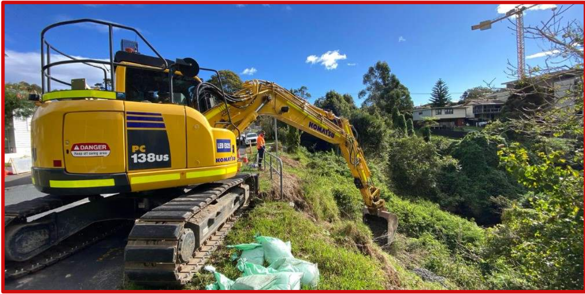
Emergency works being carried out on Whitty Road in Helensburgh, June 2024.
