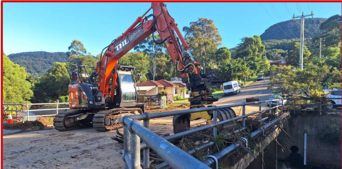
Cleanup works on Koloona Avenue, Figtree, April 2024.
