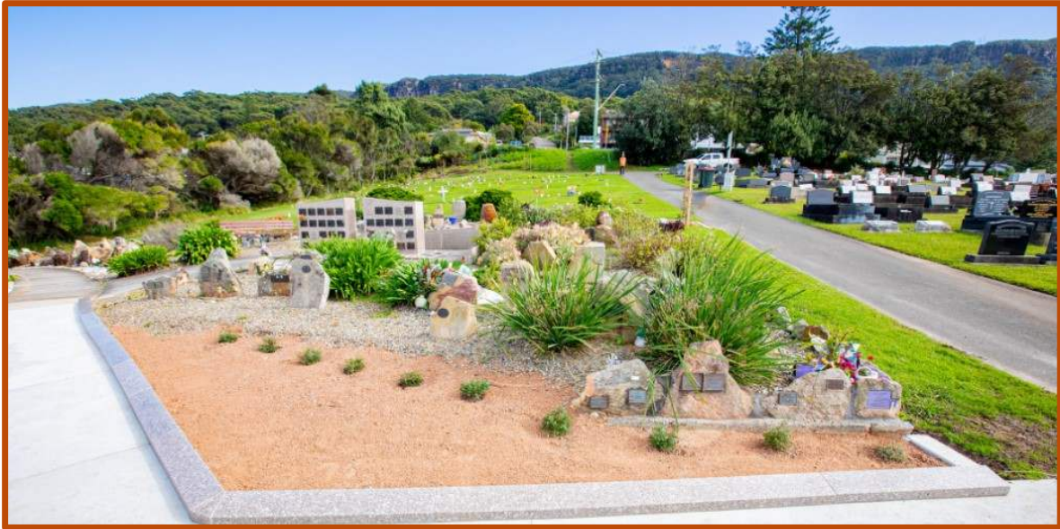
New ash walls and gardens at the Scarborough Cemetery, Scarborough. Following an extensive construction project in May 2024, there are now up to 480 new ash memorial spaces available.
