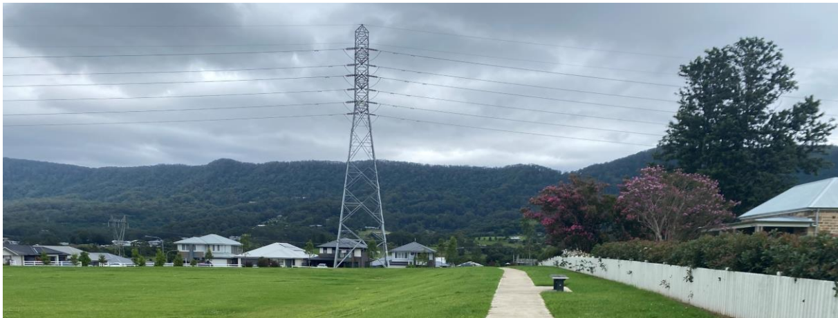
Figure 18 Site elevation of the high voltage powerline running north-south within Stane Dyke Park
