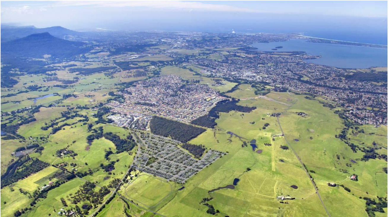
Figure 1 WDURA – aerial view looking north east
