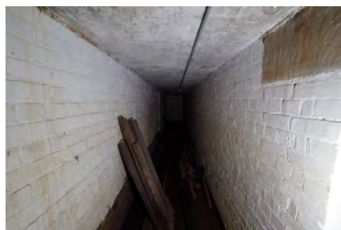
Figure 3.100 Passageway showing brick walls, concrete ceiling and a stone corner.
