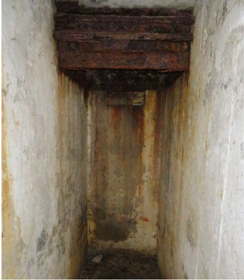
Figure 3.53 The end of one of the ventilated tunnels. It appears the vent has now been covered over.
