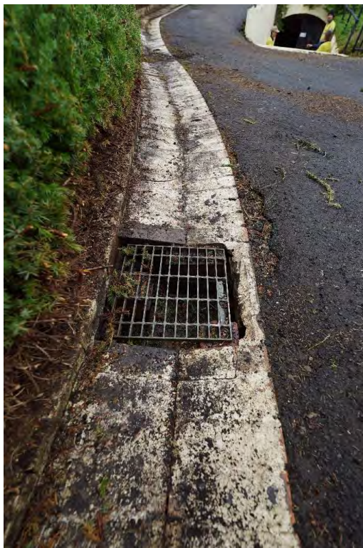
Figure 1.30 Modern drains have been installed which interface with the potentially original dish-drains. Their alignment is concealed by the asphalt surface.
