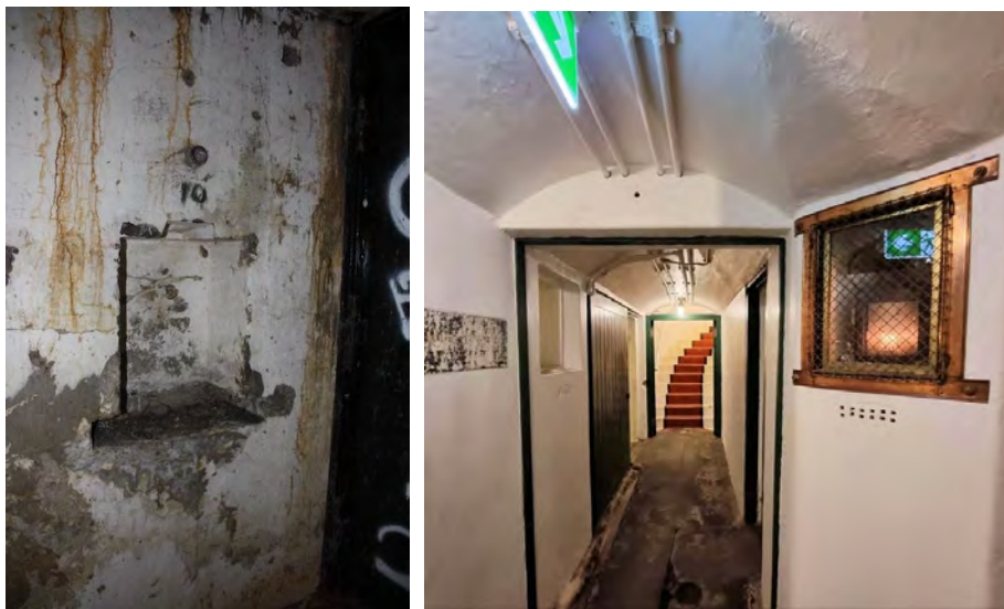
Remnants of the lantern niches which featured a safety light casing. Similar safety lights at Fort Scratchley, Newcastle.
