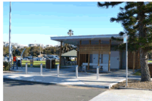
Public amenities block - clean and accessible.
