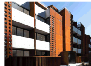
A contextually inspired medium density residential development. This project reinvigorates a prominent industrial site in Pyrmont NSW. Designed by TZG
