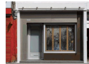
Residential shopfront conversion in a quiet main street. Front glass has a marbled pattern to create a point of interest visible from the street when lit from within at night.
