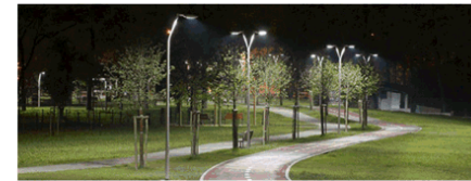
Well lit pathways, with high visibility allow for uses day and night.
