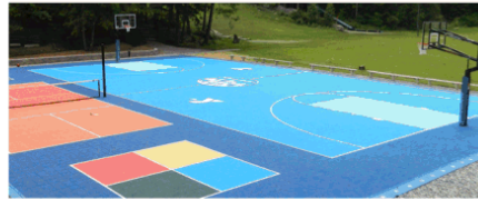
Lines could be remarked on existing court to create a multi-use court.
