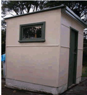
Figure 1: Bonded Asbestos (Fibro)
