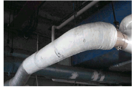
Figure 3: Friable Asbestos – Pipe Lagging
