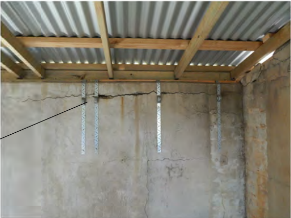
cracked wall held by braces
