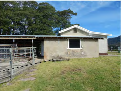
Extg broken concrete slab
