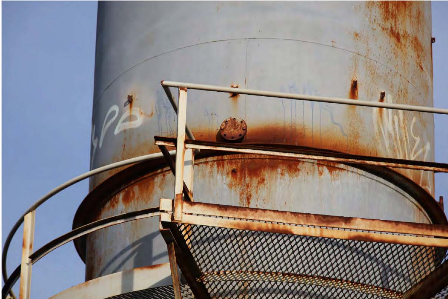
Steel chimney – significant corrosion
