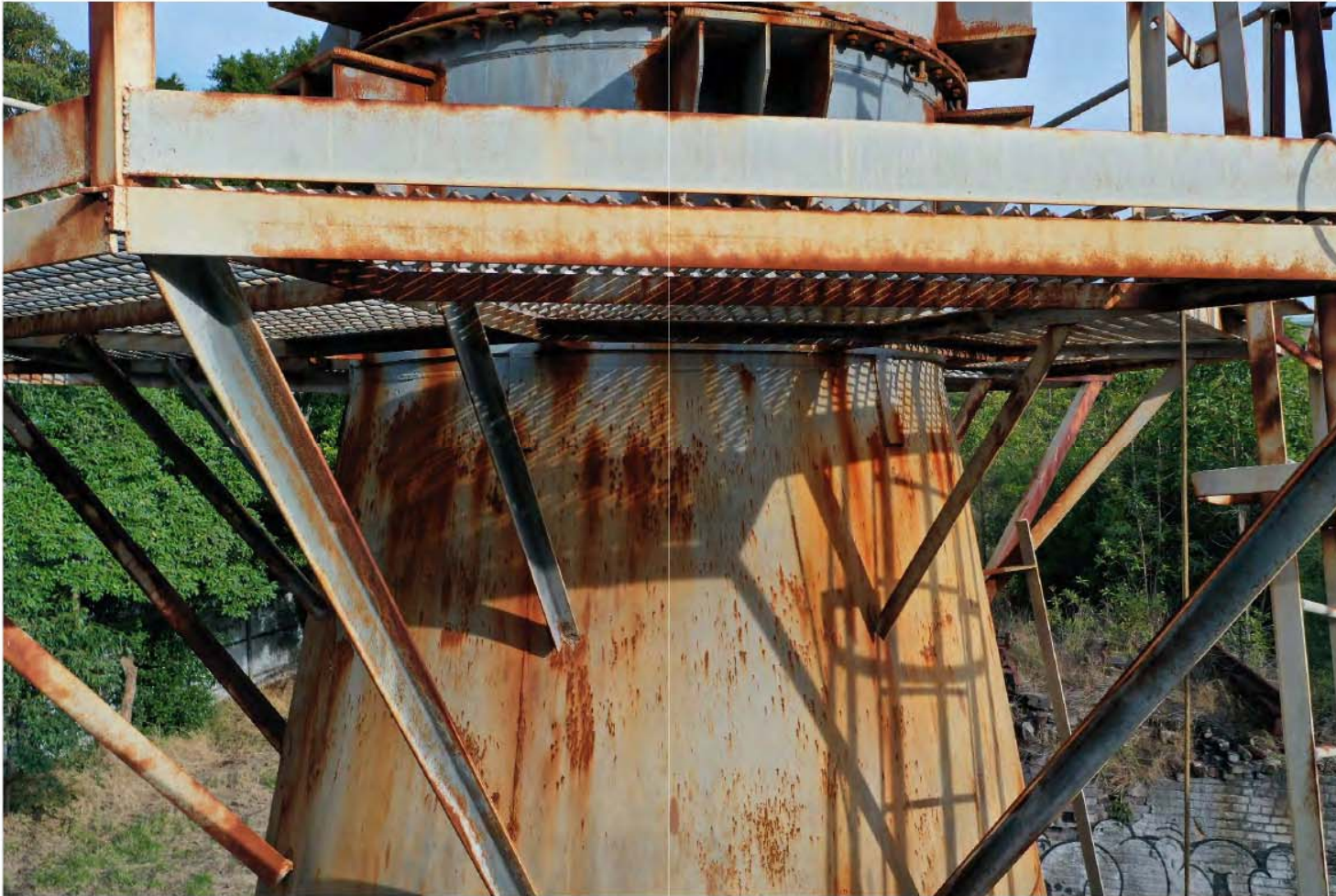
Steel chimney – significant corrosion and risk of access to platforms
