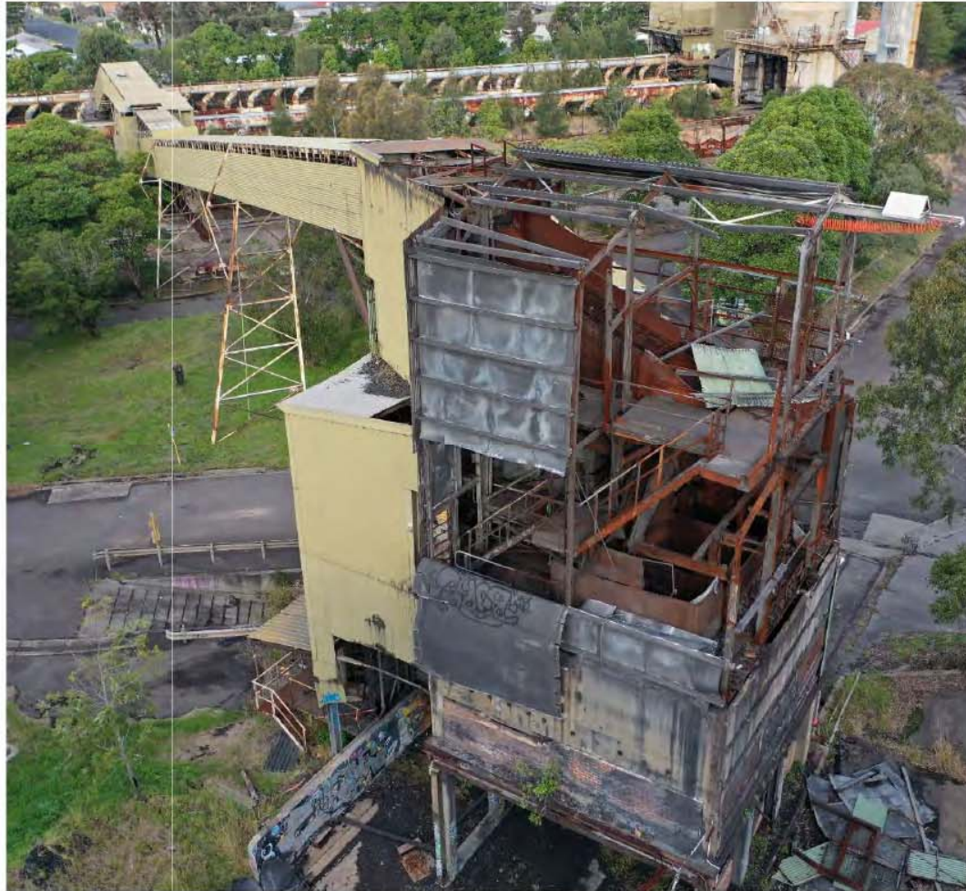
Screenhouse building – significant damage and failure of existing structural elements and cladding
