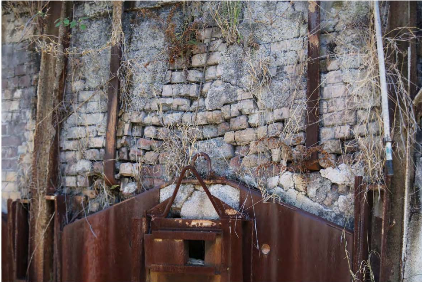
Coke ovens – slumping and failure of brickwork
