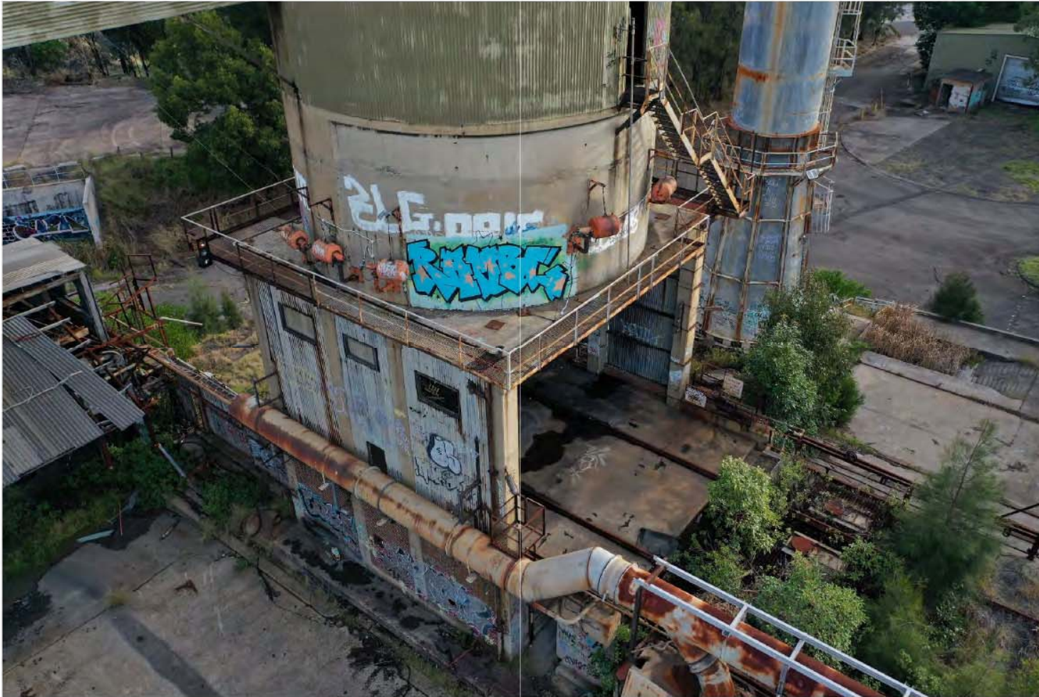
Coal bin – significant vandalism, safety risk and deterioration of fabric
