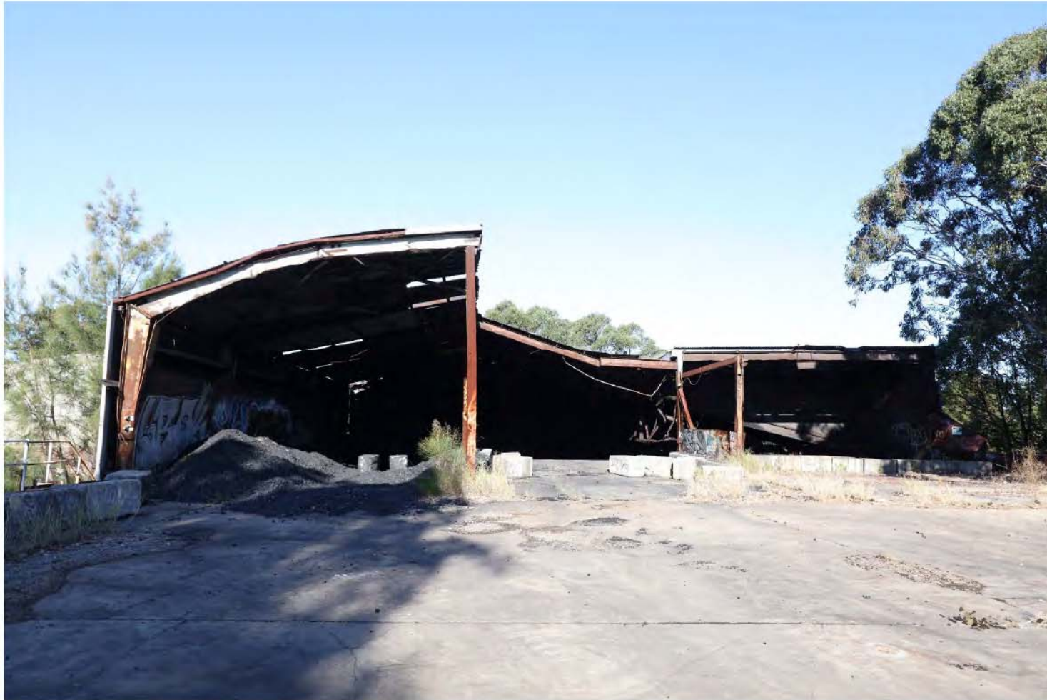
Coal bunker – significant deterioration and failure of structural support elements
