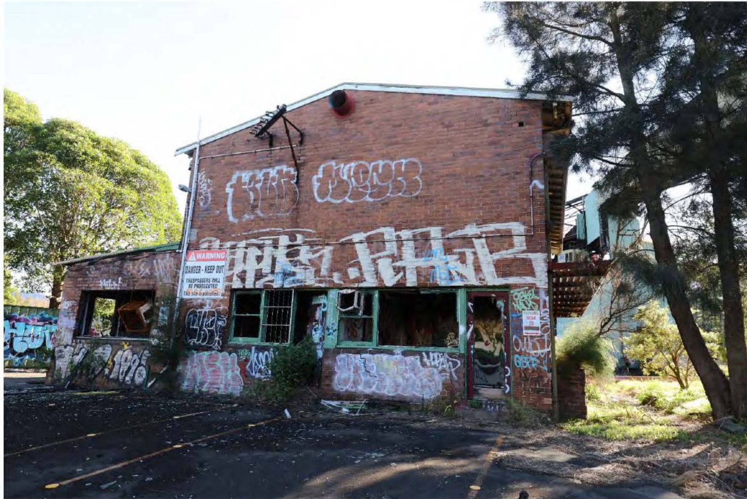
Derelict administration building with significant vandalism
