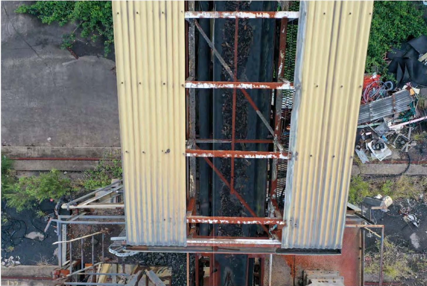
Overhead conveyor – deterioration of structural elements and significant safety issues
