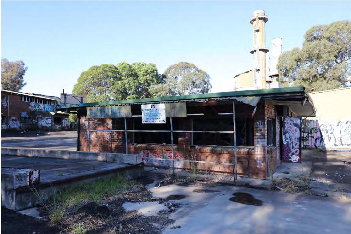
Derelict administration building with significant vandalism
