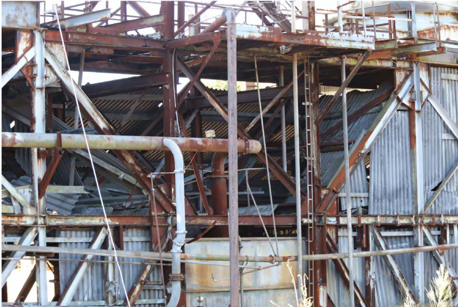
Base of quench towers – significant failure of structural elements, assessed as being at risk of major failure
