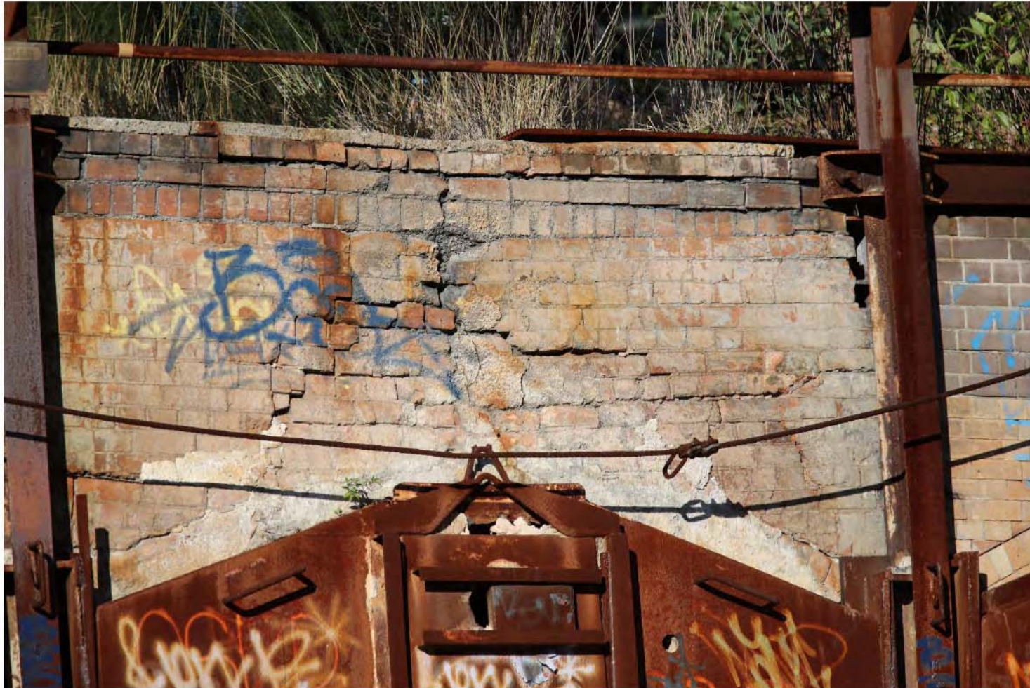
Coke ovens – slumping and failure of brickwork
