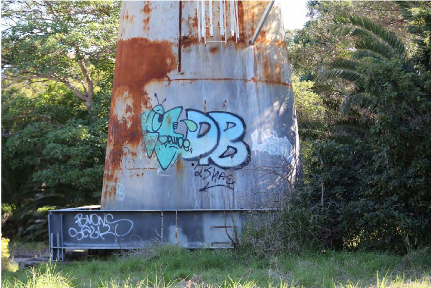
Base of steel chimney – temporary support bracing due to failure of footings
