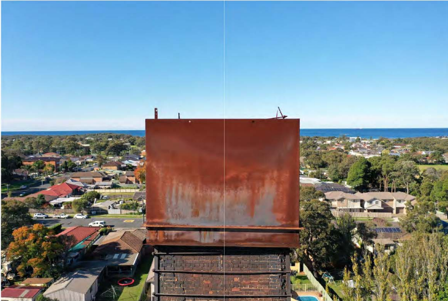
1912 Brick Chimney – significant corrosion of steel capping and failure of external brickwork
