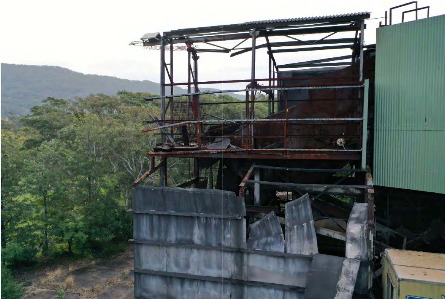
Screenhouse building – significant damage and failure of existing structural elements and cladding
