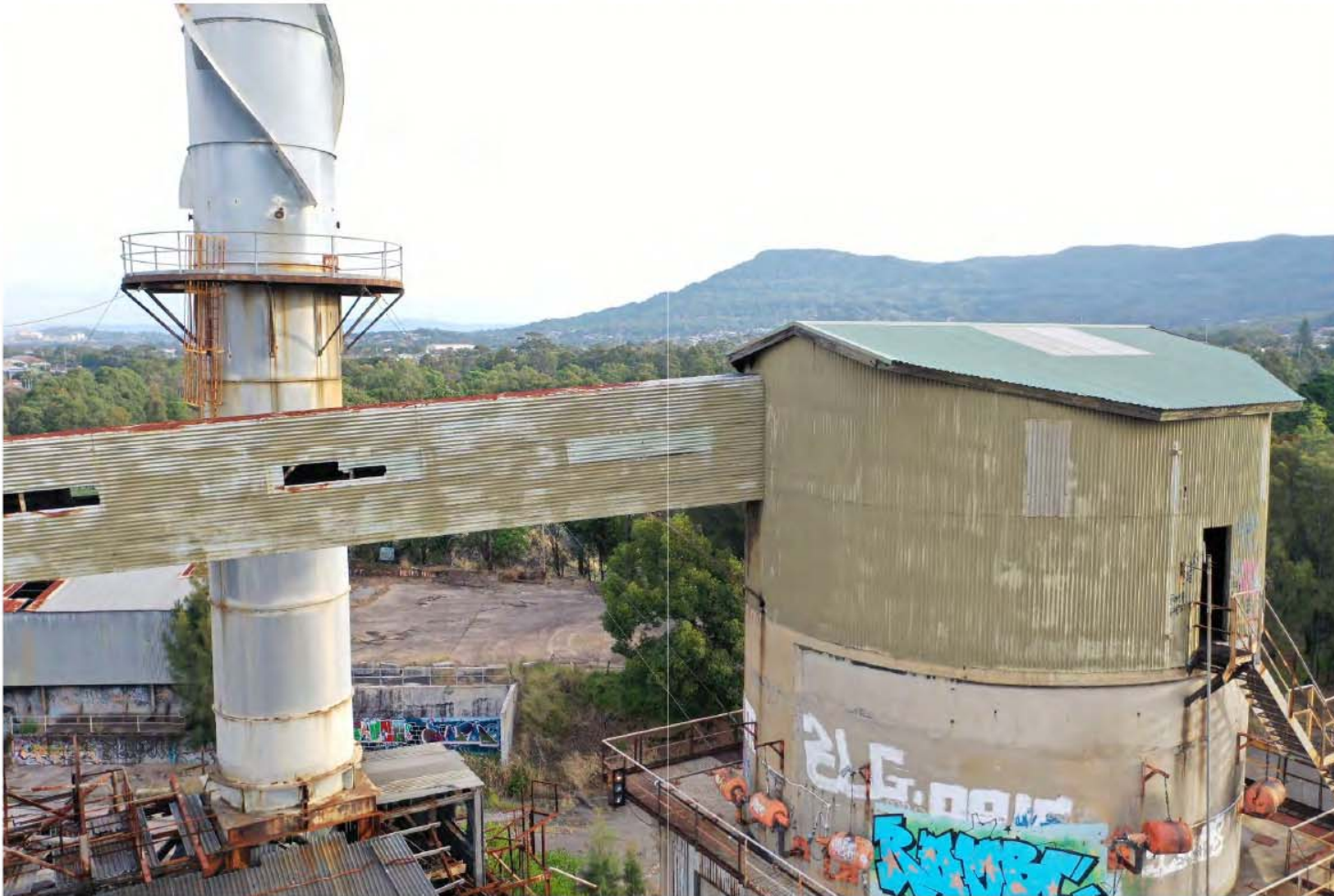
Coke conveyor and coal bin – deterioration of structural elements, cladding and significant safety issues due to access and height
