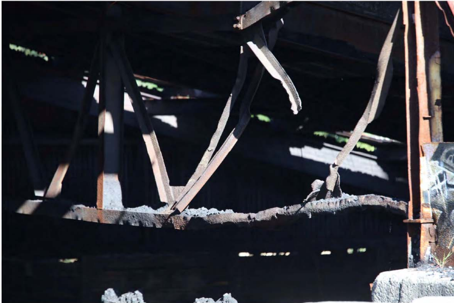
Coal bunker – failure of structural support elements
