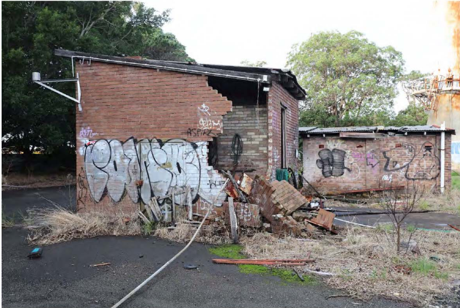
Brickies Shed – vandalism and destruction
