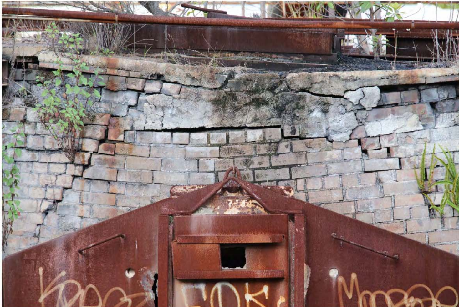
Coke ovens – slumping and failure of brickwork
