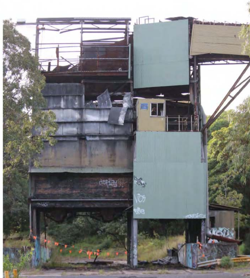
Screenhouse building – significant damage and failure of existing structural elements and cladding
