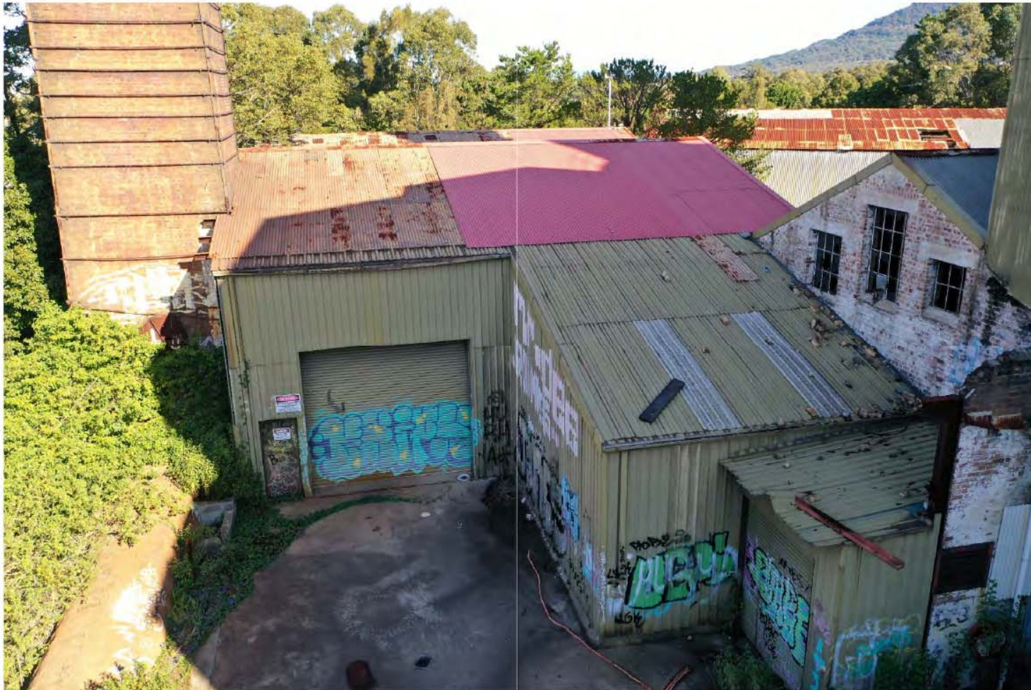
Former powerhouse building – significant vandalism and deterioration of fabric
