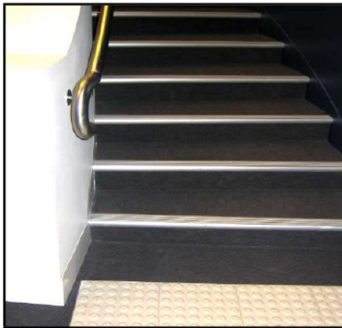
Figure 1413: Correct enclosed opaque risers with no overhangs which meet the requirements of stairways suitable for people with disabilities, under AS1428.1.
