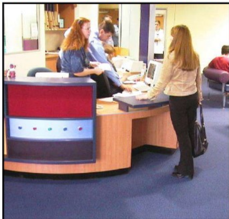
Figure 2426: (Top left) Reception counters which allow for a frontal approach with an adequate toe plate and knee space for people who use a wheelchair.
