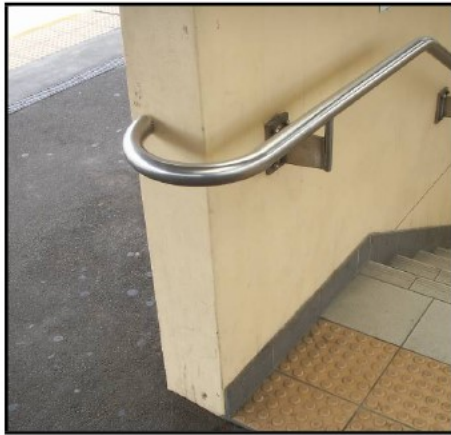
Figure 57: (Top left) Correct return of the handrail to a side wall and the required 270° top arc clearance.
