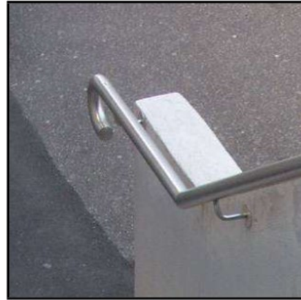
Figure 57: (Top left) Correct return of the handrail to a side wall and the required 270° top arc clearance.
