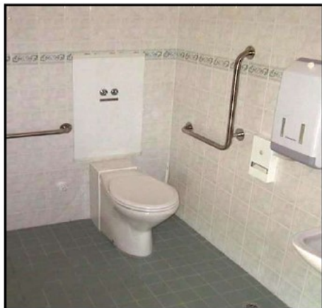
Figure 2830: The incorrect placement of the toilet paper holder too far forward of the WC pan, which forces patrons to lean excessively forward to get to the paper. This can result in patrons falling off the pan in attempting to reach the toilet holder.
