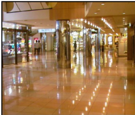
Figure 2022: (Top left) Very shiny and slippery floor surfaces which fail to meet the "R" rating, as required by AS4586 and HB197.
