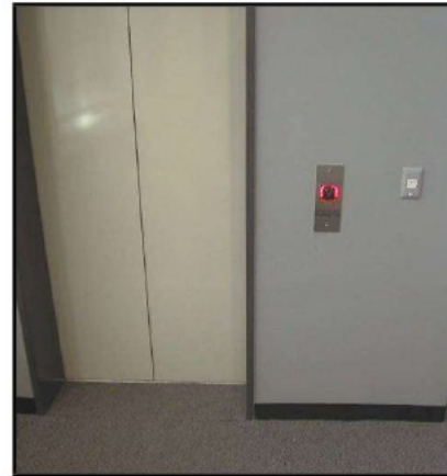
Figure 4820: (Top left) Show call buttons which comply with the requirements of AS1735.12 in terms of their placement, luminance contrast application and raised tactile and Braille which are consistently placed adjacent to each button.
