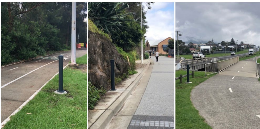
[Image: Fixed counters installed to measure usage of shared pathways]
