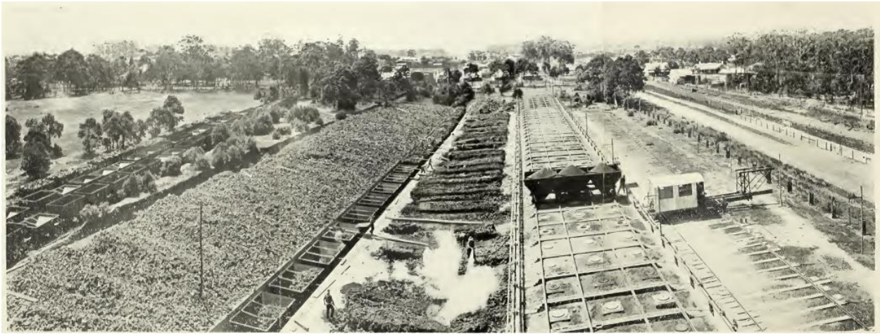
Figure 7 – Bird's-eye View of Coking Plant. The Corrimal-Balgownie Collieries, Ltd., Corrimal. Photo: LF Harper. Shows the coking process including coal delivery, charge car, push car and hand quenching in process.
