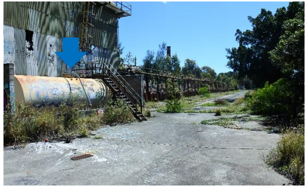
Figure 19 – Waste Oil Storage Tank
