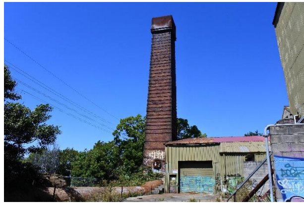
Figure 4 – View south from the C1 Coke Oven Battery.
