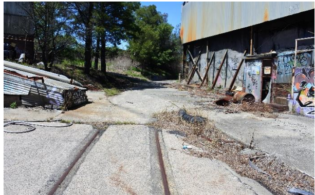
Figure 21 – View of tracks looking east.
