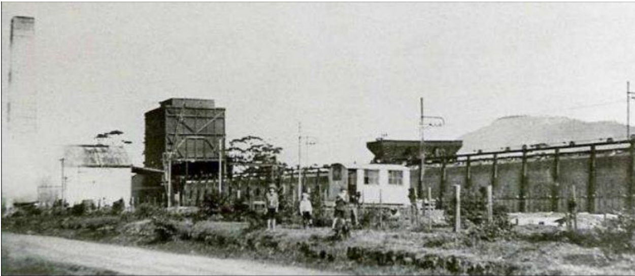
Figure 28 – Corrimal Coke Works, between 1912 and 1927. Note the original brick chimney, powerhouse, C1 batteries and pusher car and charge cars on top of the ovens
