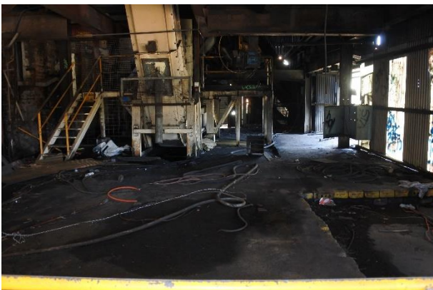
Figure 12 – View south within the grinding plant.
