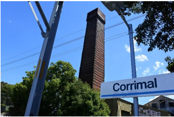
Figure 3 – View west from the Corrimal Railway Station.
