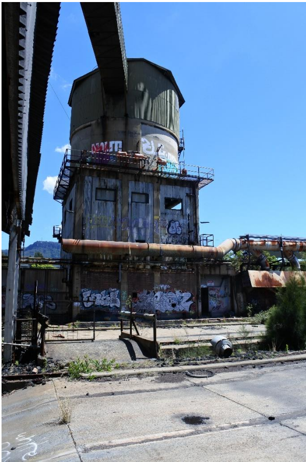
Figure 27 – View west, showing C2 Fine Coal Bin
