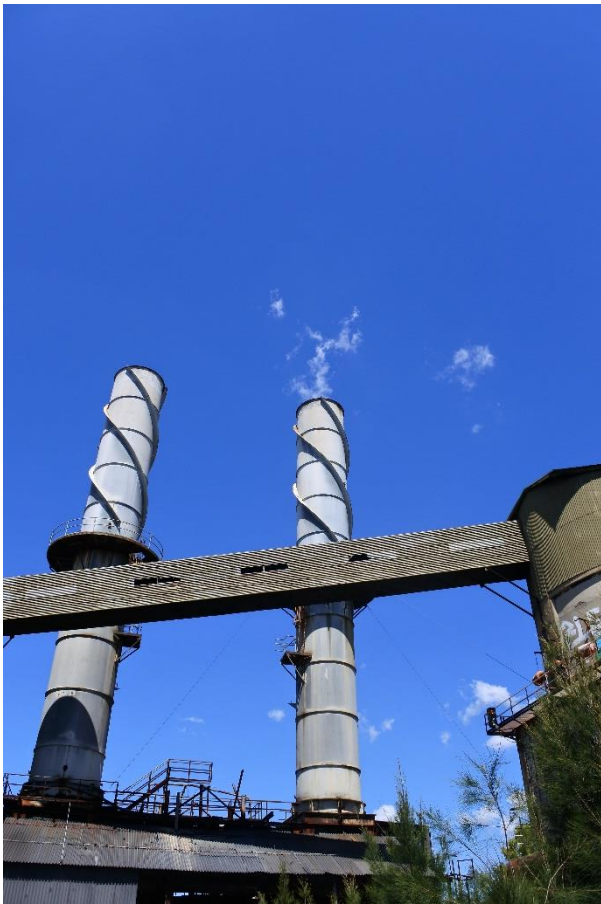
Figure 15 – View south showing quench towers.
