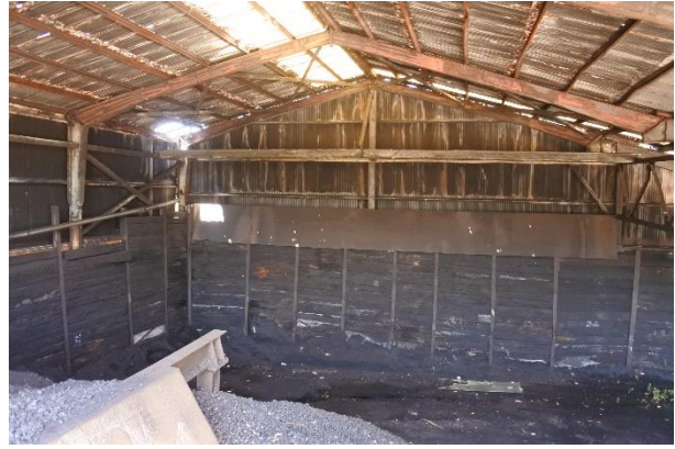
Figure 32 – View looking east inside coal storage shed.
