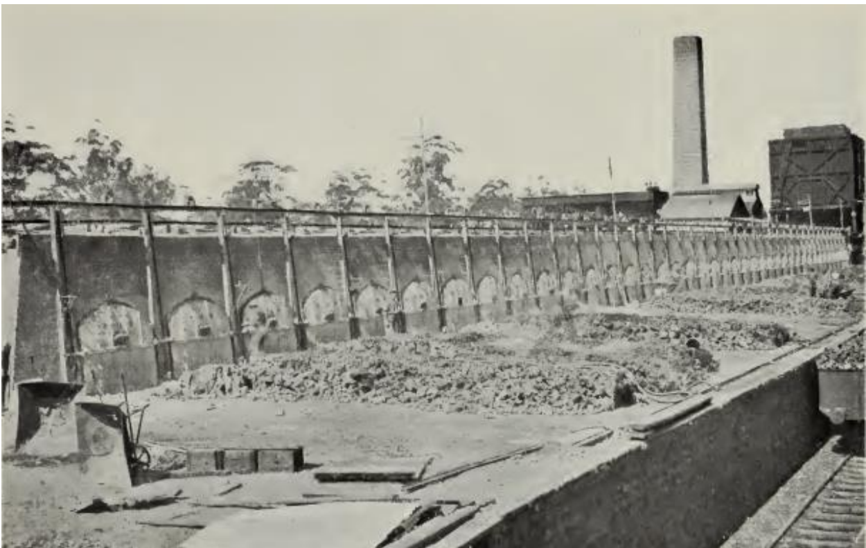
Figure 27 – Corrimal-Balgownie Co.'s Ovens at the Corrimal Coke Works, 1916.
