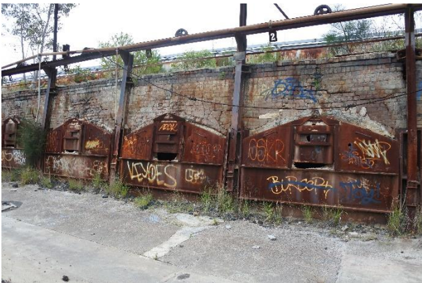
Figure 13 – View of west elevation of C2 Coke Battery, showing ovens 2, 3, 4 & 5.
