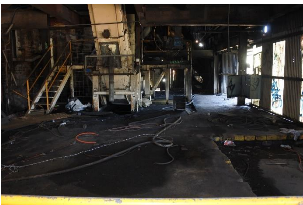
Figure 29 – View south within the grinding plant.
