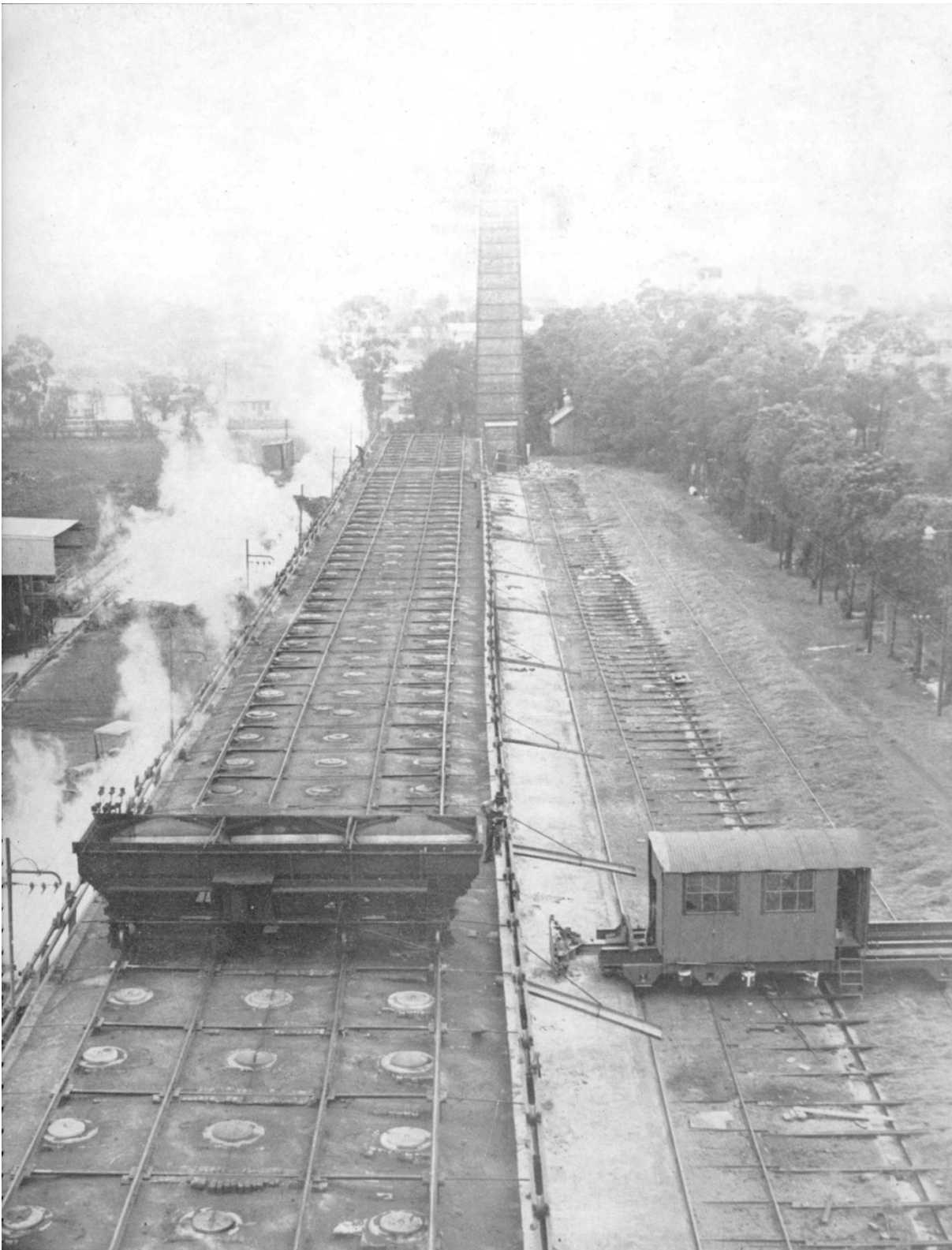
Figure 61 – Corrimal Coke Works, general view of coke ovens and quenching hearth, 1958-59.
