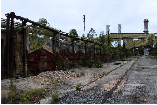
Figure 11 – View of west elevation of C2 Coke Battery.
