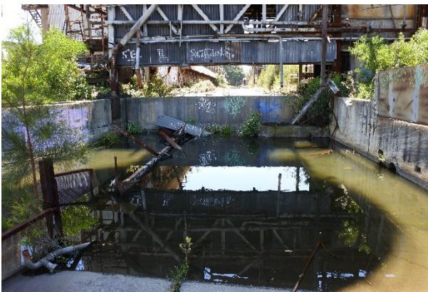
Figure 17 – View north of quench tower settling pond.
