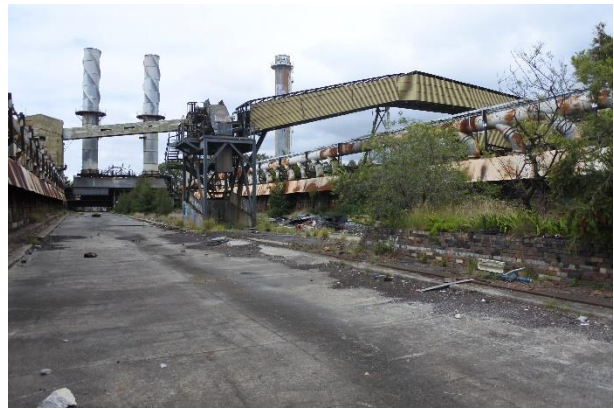
Figure 34 – View south between the two coal batteries showing the conveyor.
