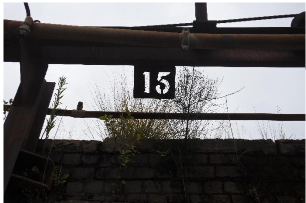
Figure 14 – Detail view of metal identifier for coke oven 15 in C2 Coke Battery.
