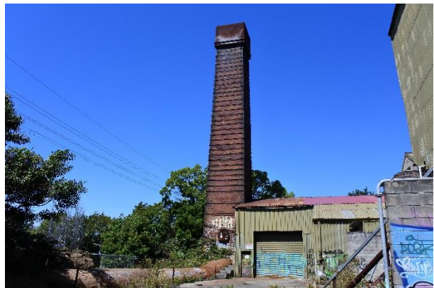
Figure 23 – View of the brick stack south from the C1 Coke Oven Battery.
