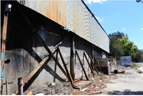
Figure 31 – View looking west, showing north elevation of coal storage shed.
