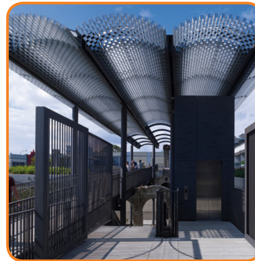
PORTION OF INTERPRETIVE ELEMENTS REFERENCING COKE OVEN ELEMENTS
