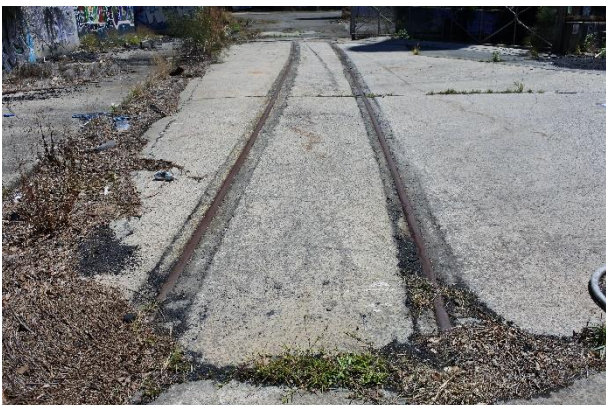
Figure 47 – View of tracks looking west.
