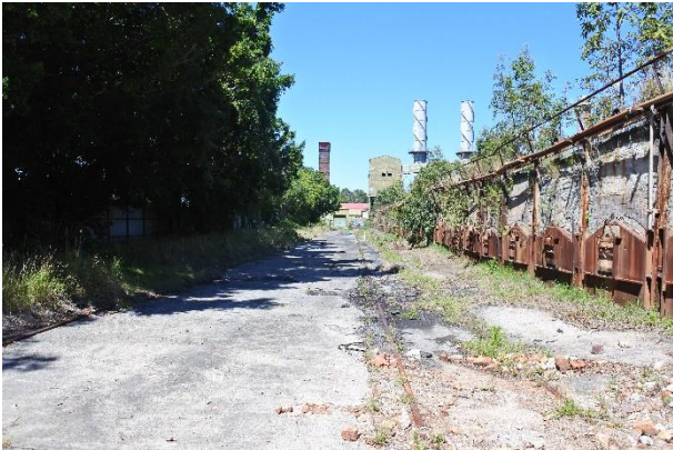
Figure 75 – View south within site, along the C1 Coke Oven Battery.
