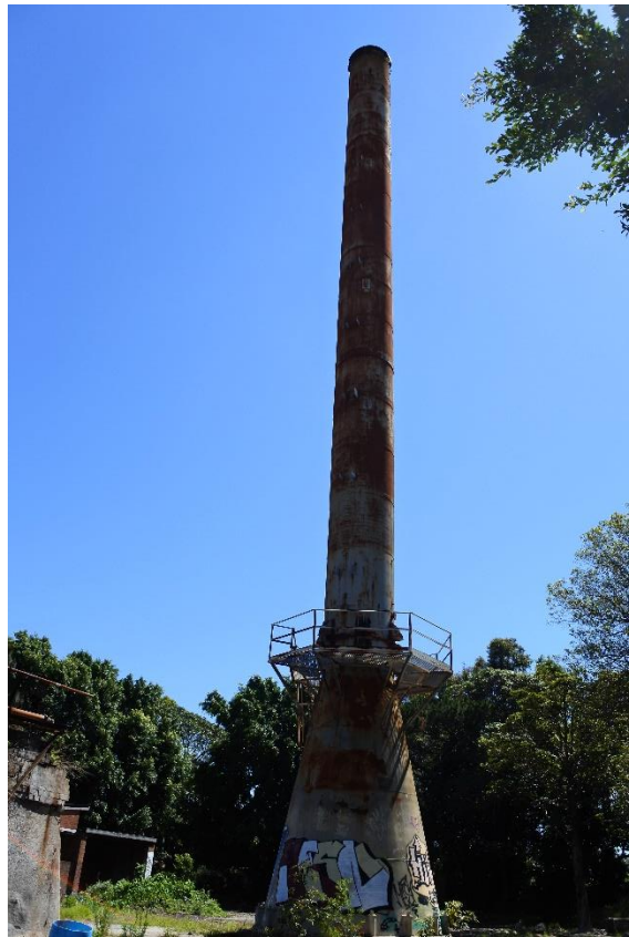
Figure 20 – Detail view of C1N stack.
