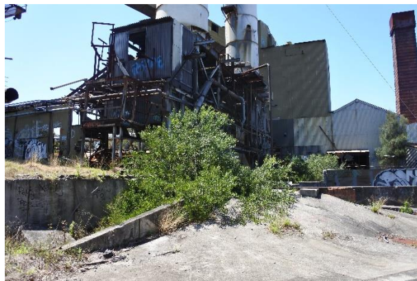
Figure 18 – View east showing structure and surrounds of quench tower base.
