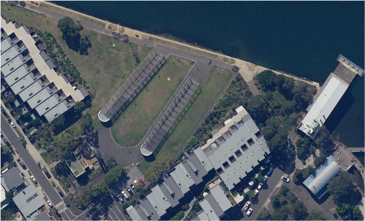
Figure 24 – Building footprint interpretation, former, Glebe Incinerator, Sydney.
