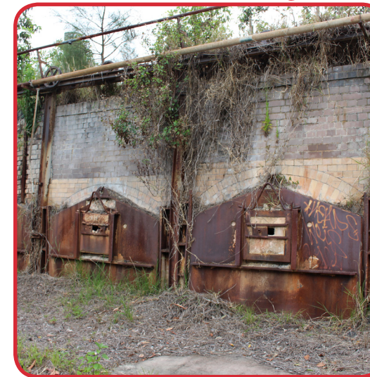
PORTION OF RECONSTRUCTION/ IN SITU RETENTION OF COKE OVENS
