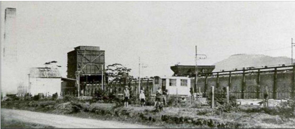
Figure 59 – Corrimal Coke Works 2 / Broadhurst Photo, between 1912 and 1927. Note the original brick chimney, power house, C1 batteries and pusher car and charge cars on top of the ovens
