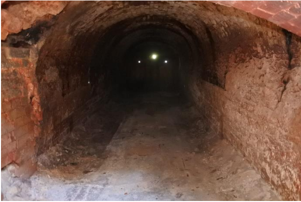
Figure 7 – View within an oven, looking west.
