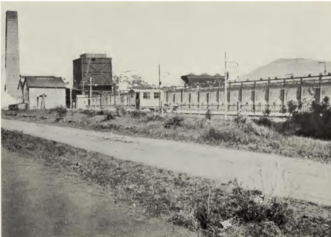
Figure 57 – Corrimal-Balgownie Co.'s Ovens, Corrimal.
