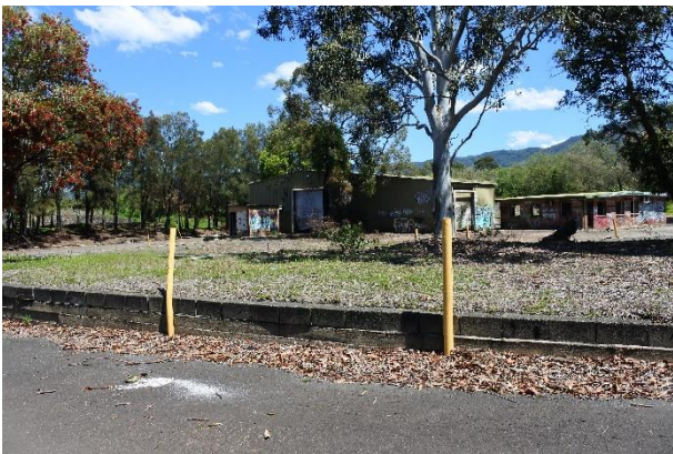
Figure 41 – Weighbridge/Crib Room and Maintenance Workshop, looking west.
