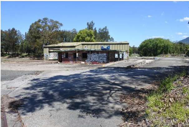
Figure 39 – Weighbridge/Crib Room and Maintenance Workshop (behind) looking south.
