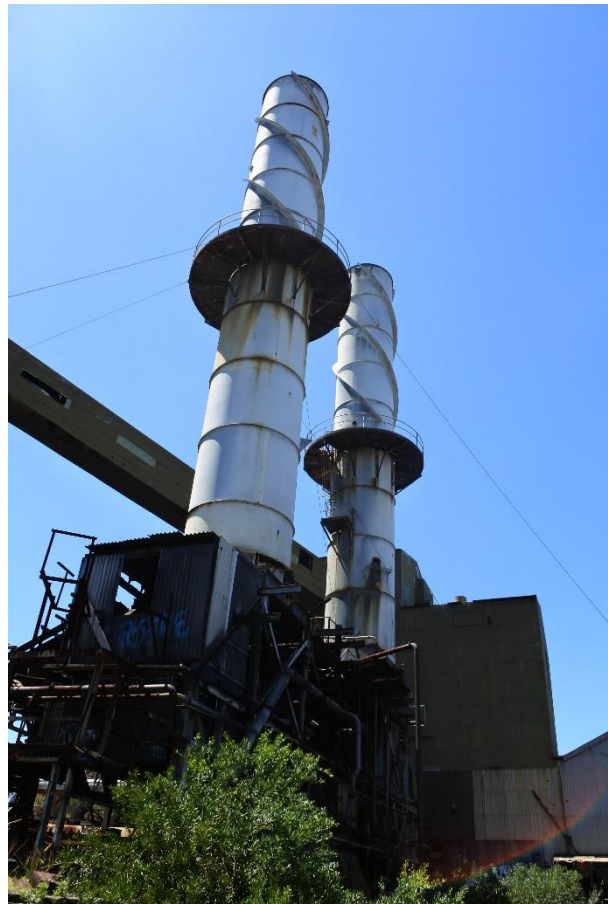
Figure 16 – View east showing quench towers and structures.
