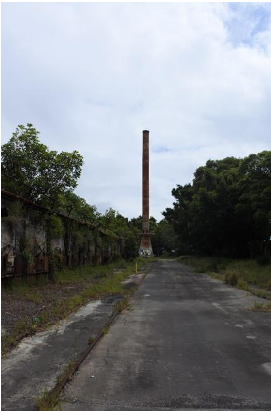
Figure 19 – View north showing C1N stack.
