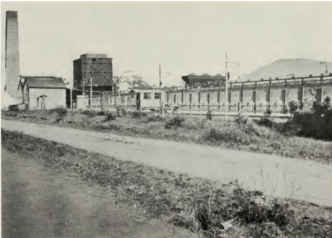
Figure 9 – Corrimal-Balgownie Co.'s Ovens, Corrimal.
