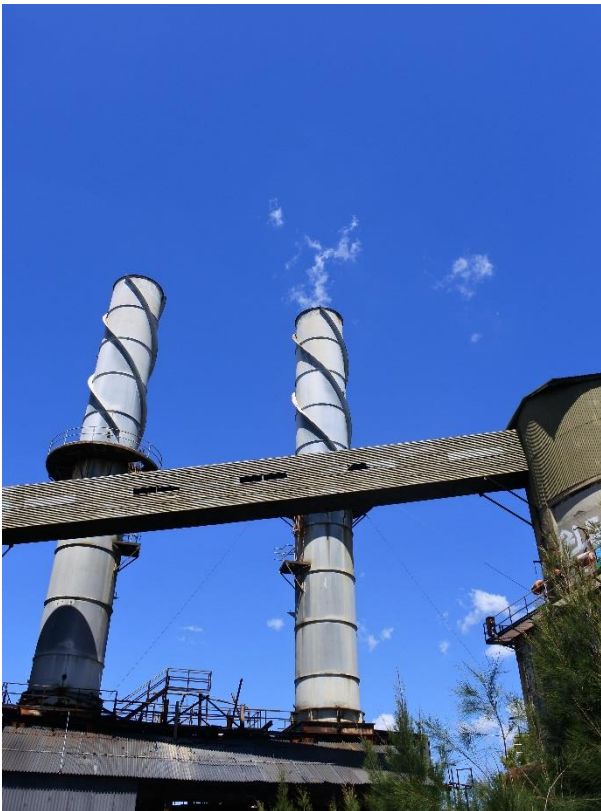
Figure 10 – View south showing quench towers.
