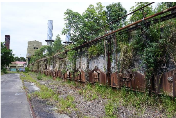
Figure 5 – View looking south of east elevation of C1 Coke Ovens.
