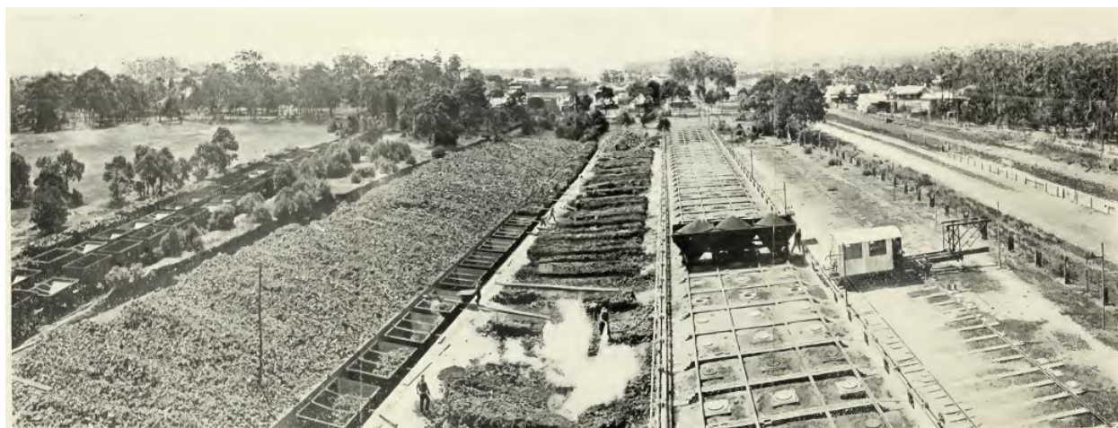
Figure 55 – Bird's-eye View of Coking Plant. The Corrimall-Balgownie Collieries, Ltd., Corrimall. Photo: LF Harper. Shows the coking process including coal delivery, charge car, push car and hand quenching in process.
