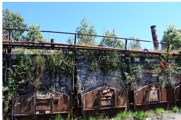
Figure 6 – View of east elevation of C1 Coke Ovens - 31,32 & 33.
