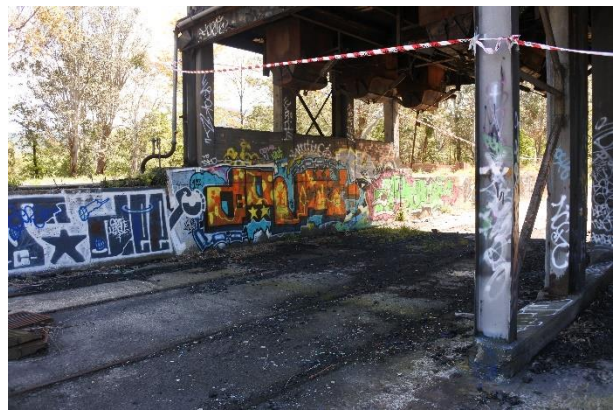
Figure 36 – View under the coke screen house showing railway line remnants.
