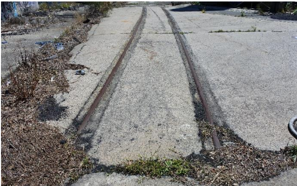
Figure 20 – View of tracks looking west.
