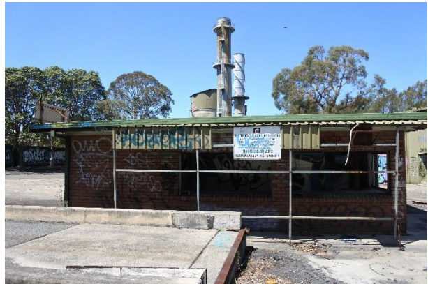
Figure 40 – Weighbridge/Crib Room, looking east.
