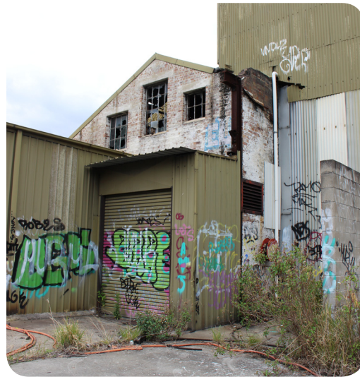
REMNANT POWERHOUSE AND REMNANT 1912 POWERHOUSE GABLE WALL
