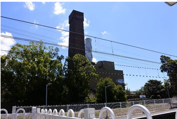
Figure 79 – View west from Corrimal Station, prominent view of Brick Stack.
