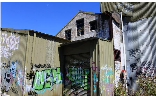
Figure 24 – View of the remnant wall of the former power house.
