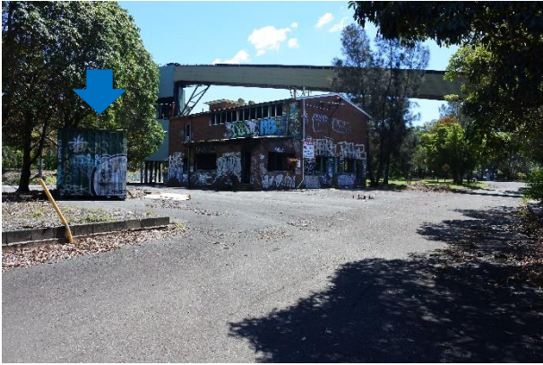
Figure 43 – Oil Storage Tank
