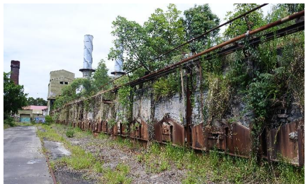
Figure 25 – View looking south of east elevation of C1 Coke Ovens.
