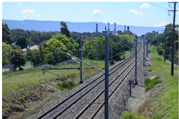
Figure 80 – View north along the South Coast Line from Towradgi Road railway overbridge.
