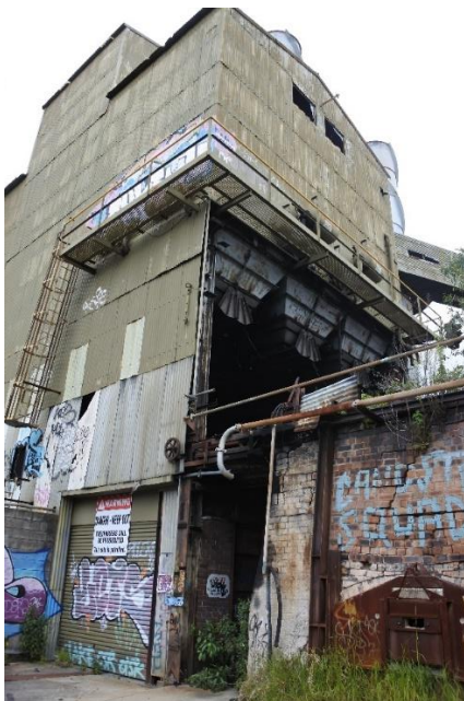
Figure 25 – View west, showing C1 Fine Coal Bin
