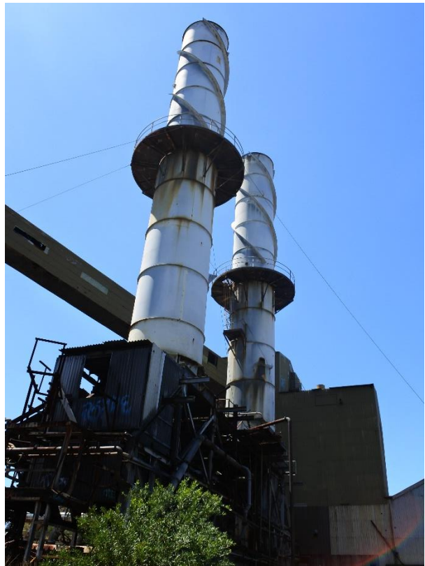
Figure 11 – View east showing quench towers and structures.
