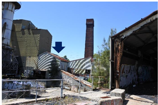
Figure 13 – View looking east showing grinding plant.
