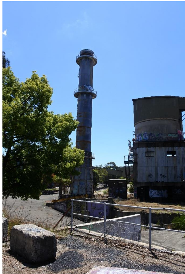
Figure 28 – View north, showing C2 Fine Coal Bin
