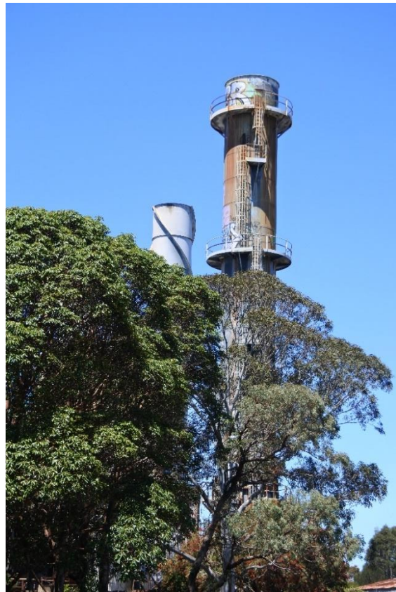
Figure 24 – View east showing C2S stack with one of the quench towers to the left.
