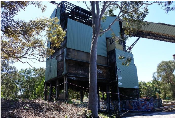
Figure 33 – View of south and west elevations of coke screen house and conveyor.
