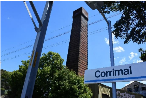
Figure 22 – View of the brick stack looking west from the Corrimal Railway Station.
