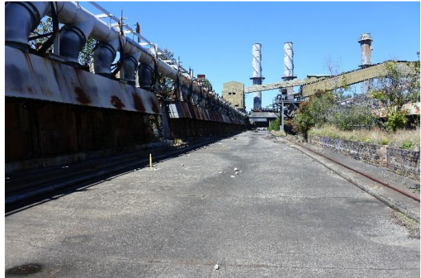
Figure 76 – View south along the west elevation of the C1 Coke Oven Battery to the Quench Towers.
