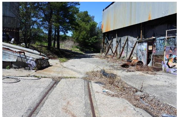
Figure 48 – View of tracks looking east.
