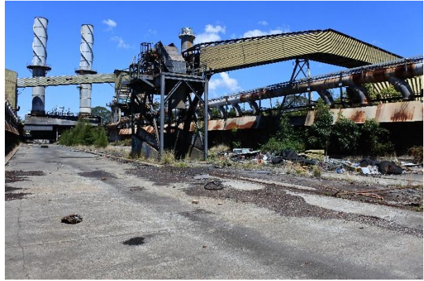
Figure 9 – View of east elevation of C2 Coke Battery.
