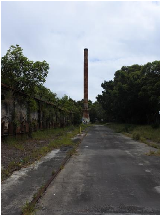
Figure 14 – View north showing C1N stack.
