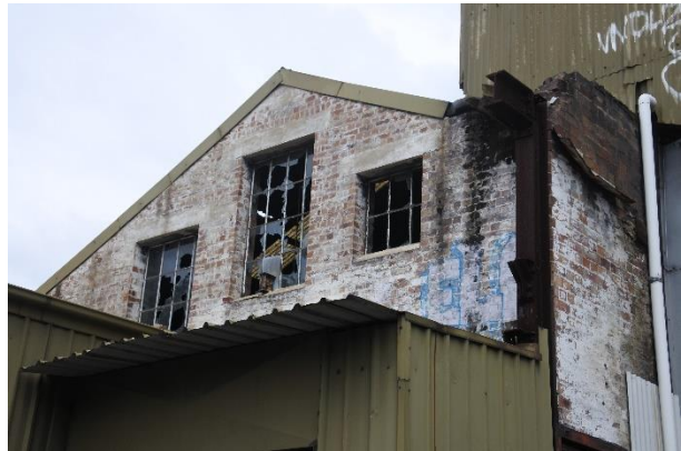
Figure 10 – Detail view of the remnant of the former power house.
