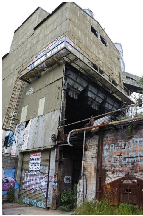
Figure 17 – View west, showing C1 Fine Coal Bin.
