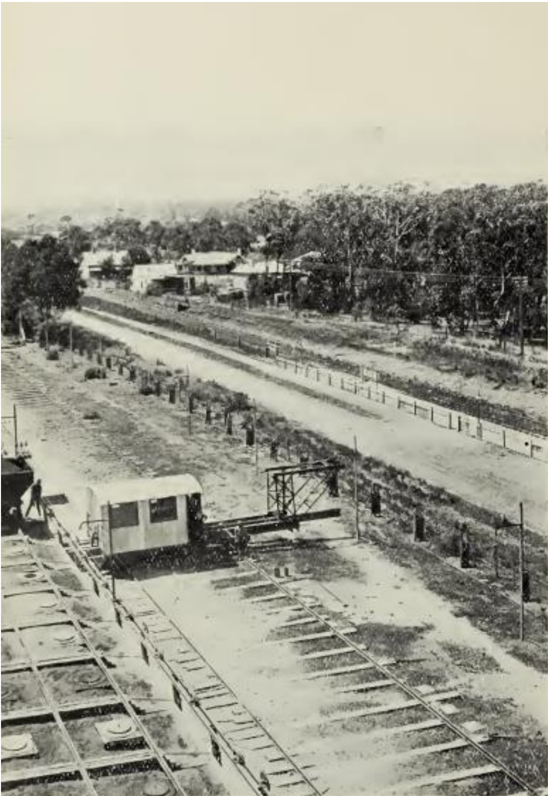
Figure 8 – Another view of Coking Plant. The Corrimal-Balgownie Collieries, Ltd., Corrimal. Shows the coking process including coal delivery, charge car, push car and hand quenching in process.
