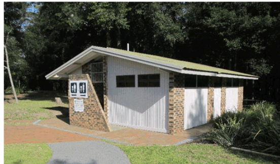
Toilet block at Mt Keira
