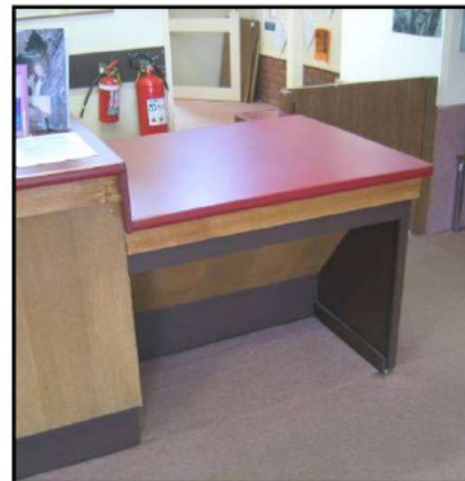
Figure 2426: (Top left) Reception counters which allow for a frontal approach with an adequate toe plate and knee space for people who use a wheelchair.
