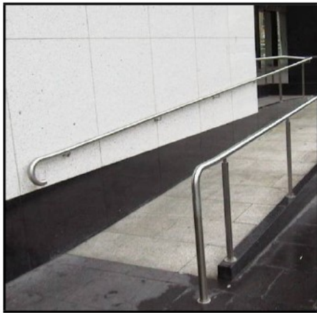
Figure 43: (Top left) Correct application of returning the handrail down and back onto itself to form 180° return onto a post. The handrails also provide clearances on the top 270° arc of the handrail and the 15mm directly under the handrail to allow for uninterrupted transition along the full length of the handrail for fingers and thumbs.
