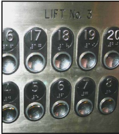
Figure 4820: (Top left) Show call buttons which comply with the requirements of AS1735.12 in terms of their placement, luminance contrast application and raised tactile and Braille which are consistently placed adjacent to each button.
