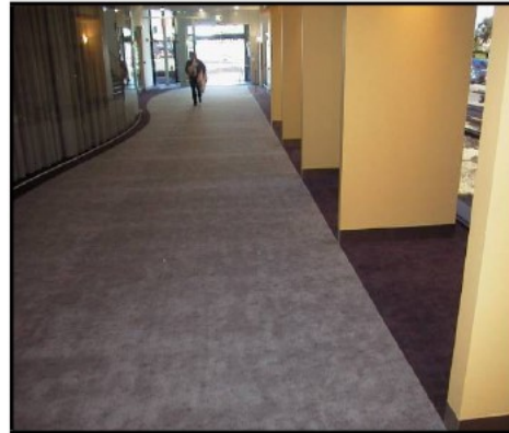
Figure 2224: (Top left) Show floor surfaces which meet the “R” rating under AS4586 and HB197.
