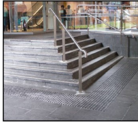
Figure 4214: (Top left) TGSIs which fail to comply with the specifications of AS 1428.4 since they fail to provide the required luminance contrast. Under AS1428.4, a minimum of 30% luminance contrast is required for TGSIs, compared to the surrounding floor/ground surface. These photographs also show other non-compliant features such as the handrails and the lack of colour contrasting nosings.
