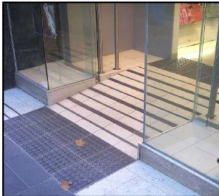
Figure 4719: A threshold ramp with an automatic door into a retail premises which complies with the BCA and AS1428.1 (without the need for a landing area).
