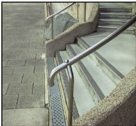
Figure 35: (Top left) Handrails which do not comply with the specifications of AS1428.1 for handrails on stairs suitable for people with a disability since the handrails fail to return to a side wall or downwards and back on themselves at 180°.
