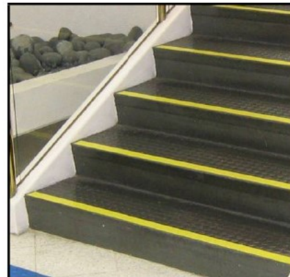
Figure 79: (Top left) The correct minimum luminance contrast and depth of treatment on the nosings of the treads / goings.
