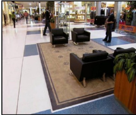
Figure 2224: (Top left) Show floor surfaces which meet the “R” rating under AS4586 and HB197.
