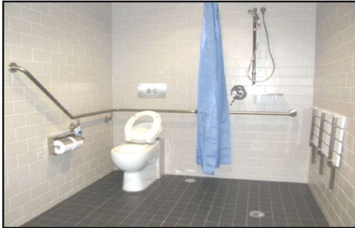
Figure 2628: Correct placement of toilet and shower fittings as per the requirements of AS1428.1. Note: The toilet roll holders are placed below the grab rail, to ensure people who use a wheelchair are able to rise off the pan and transfer back onto their wheelchair unencumbered.
