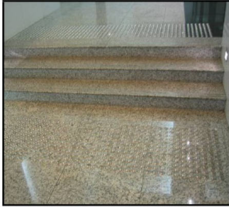
Figure 4214: (Top left) TGSIs which fail to comply with the specifications of AS 1428.4 since they fail to provide the required luminance contrast. Under AS1428.4, a minimum of 30% luminance contrast is required for TGSIs, compared to the surrounding floor/ground surface. These photographs also show other non-compliant features such as the handrails and the lack of colour contrasting nosings.
