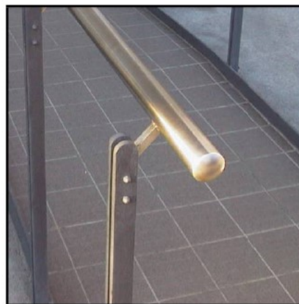
Figure 35: (Top left) Handrails which do not comply with the specifications of AS1428.1 for handrails on stairs suitable for people with a disability since the handrails fail to return to a side wall or downwards and back on themselves at 180°.
