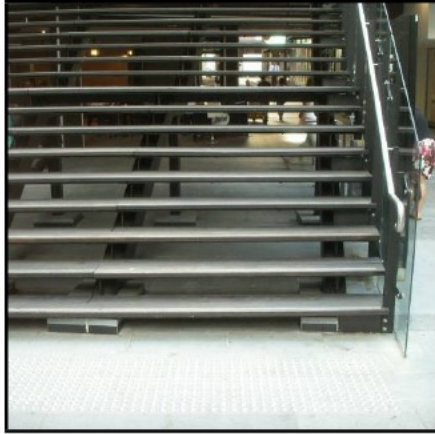
Figure 911: (Top left) Open risers and light sources coming from behind the stairway. Any person with a walking stick may lose their footing if their stick slipped through the stairway openings.
