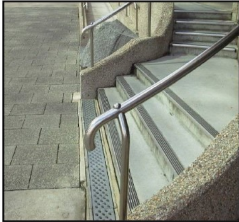
Figure 5: (Top left) Handrails which do not comply with the specifications of AS1428.1 for handrails on stairs suitable for people with disability since the handrails fail to return to a side wall or downwards and back on themselves at 180°.
