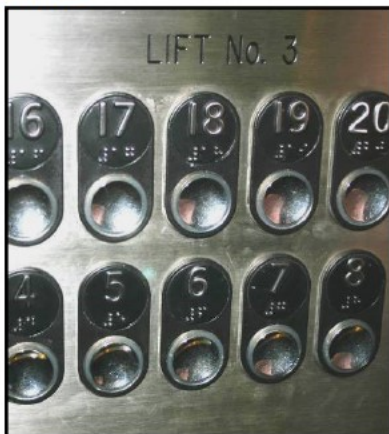
Figure 20: (Top left) Show call buttons which comply with the requirements of AS1735.12 in terms of their placement, luminance contrast application and raised tactile and Braille which are consistently placed adjacent to each button.
