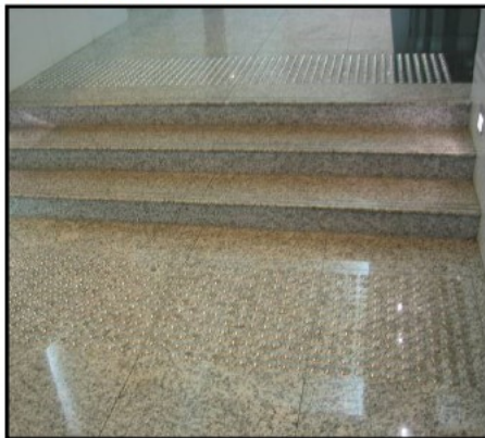
Figure 14: (Top left) TGSIs which fail to comply with the specifications of AS 1428.4 since they fail to provide the required luminance contrast. Under AS1428.4, a minimum of 30% luminance contrast is required for TGSIs, compared to the surrounding floor/ground surface. These photographs also show other non-compliant features such as the handrails and the lack of colour contrasting nosings.
