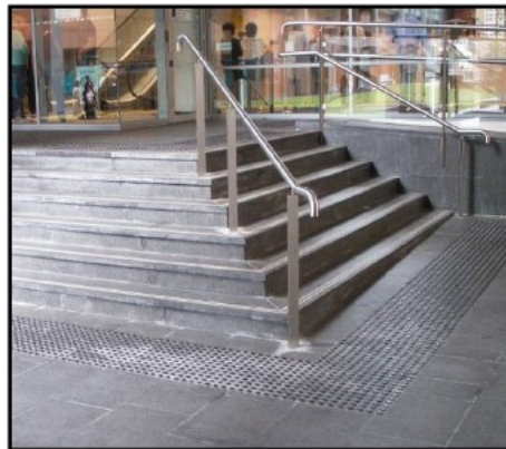
Figure 14: (Top left) TGSIs which fail to comply with the specifications of AS 1428.4 since they fail to provide the required luminance contrast. Under AS1428.4, a minimum of 30% luminance contrast is required for TGSIs, compared to the surrounding floor/ground surface. These photographs also show other non-compliant features such as the handrails and the lack of colour contrasting nosings.
