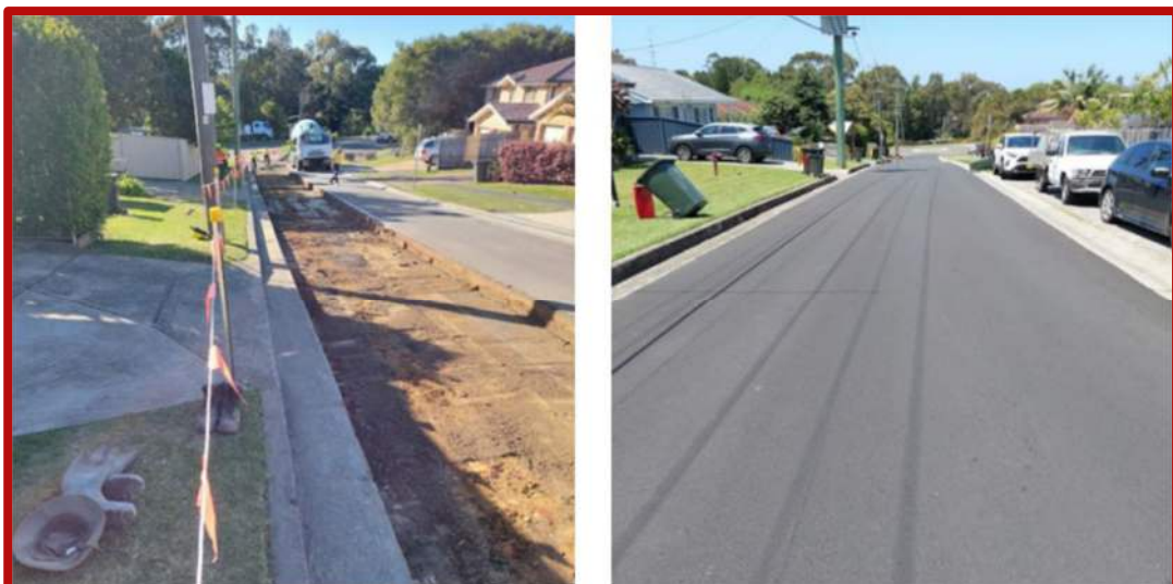
Road reconstruction work at Gahans Lane, Woonona.
