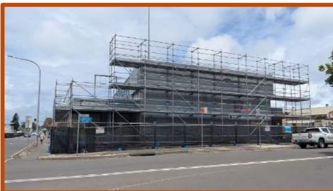
Demolition commenced at the Southern Suburbs Community Centre and Library site.
