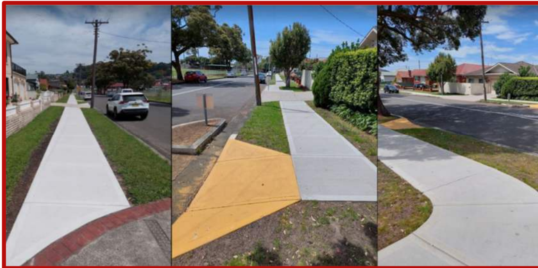
New footpath works at Union Street, Coniston.
