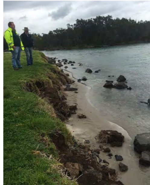
Figure 2-5 Examples of Erosion near Reddall Reserve
