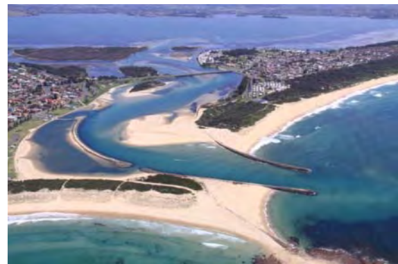
2009: trained entrance, with twin breakwaters and southern training wall fixing the entrance opening position.
