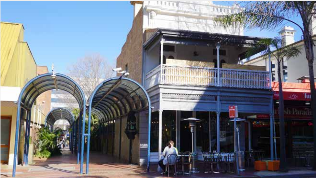
Ethel Hayton Walk increases pedestrian connectivity in Lower Crown Street
