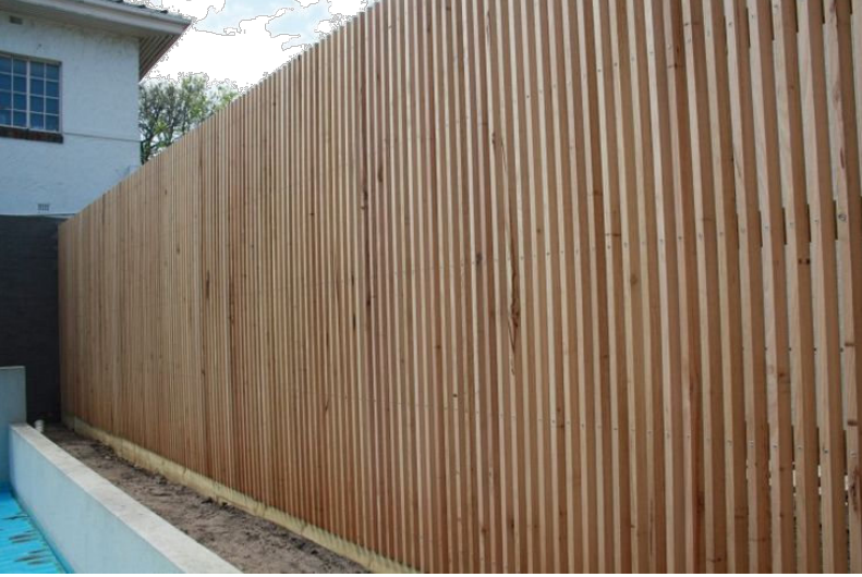
1800MM HIGH TIMBER BATTEN FENCE + GATES
