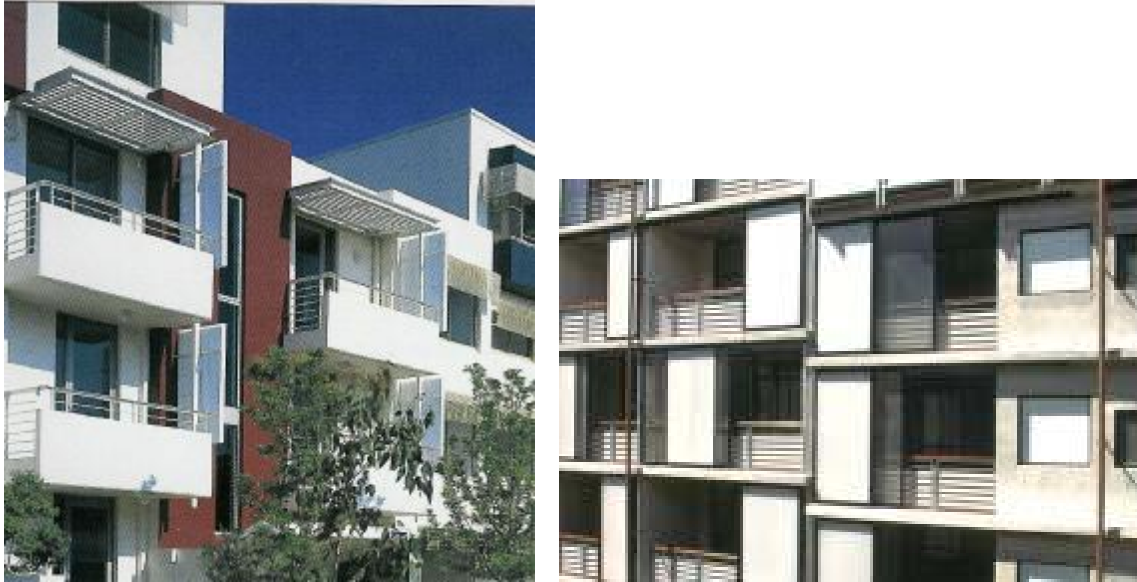
Figure 5: Examples of balcony screening and climate control elements. Reference: Residential Flat Design Code
