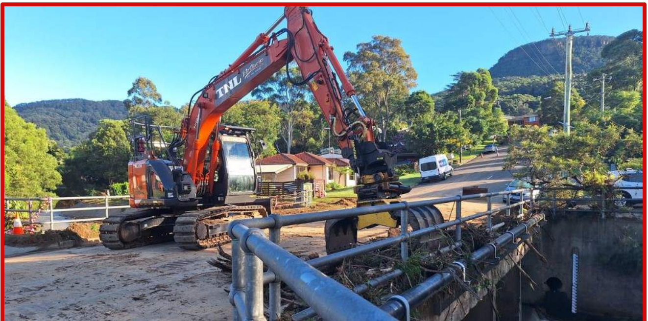
Cleanup works on Koloona Avenue, Figtree, April 2024.
