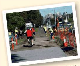
Construction of Puckey's shared pathway
