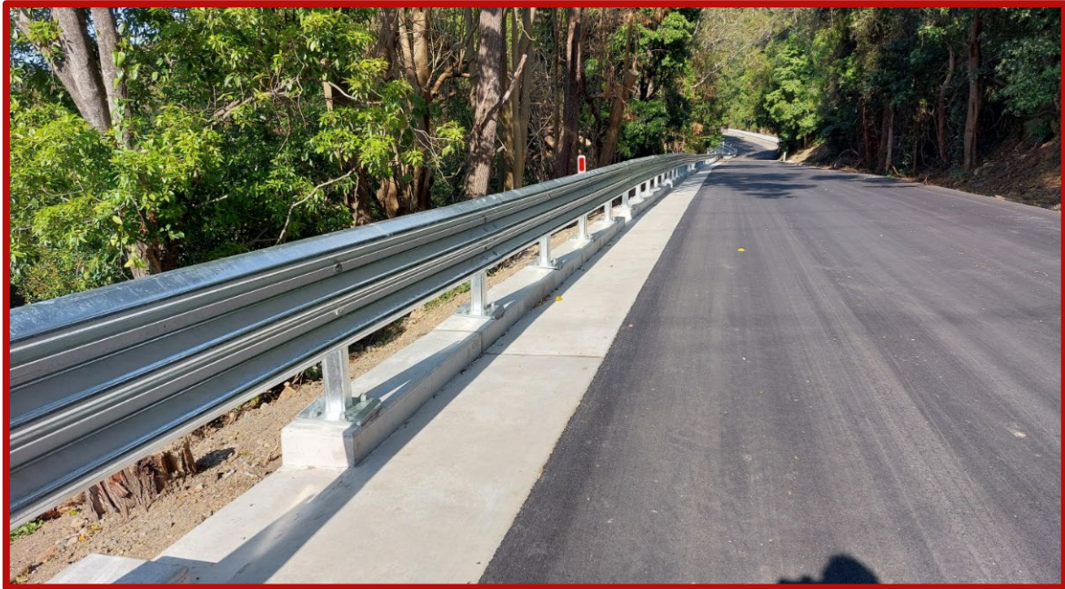
Harry Graham Drive, a key east-west link reopened after extensive works to stabilise and repair the road.
