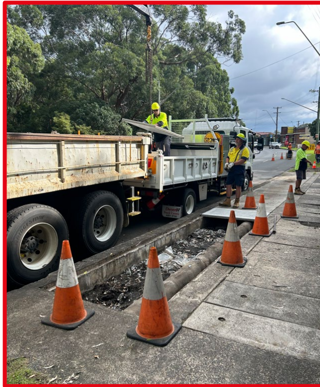
Council crew carrying out maintenance at Angels Bridge, Corrimal.
