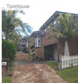
NAME: Townhouse at Gilmore (1980s) ADDRESS: 8 Gilmore St INFO: 2 storeys, 3 units, 863.2 m2 site CATEGORY: Residential DENSITY: 35 units/Ha (MEDIUM) PRINCIPLES: U1 U2 U3 U5
