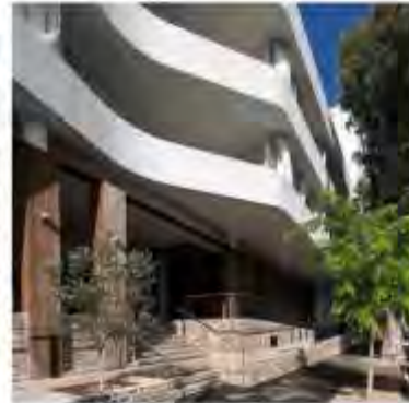
Example of flood resilient design that achieves pedestrian amenity ( www.sjb.com.au , 2017)
