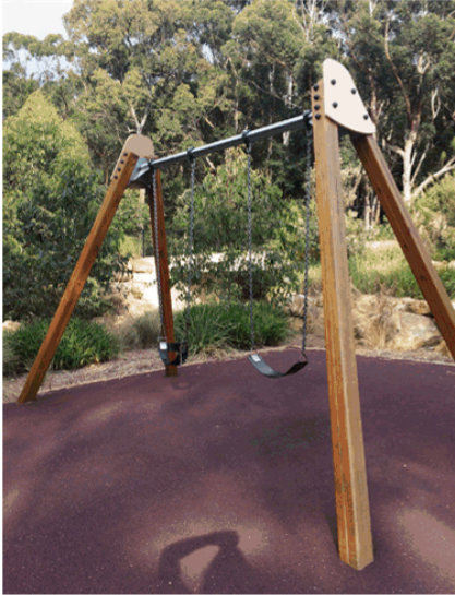
Wet pour surface treatment under swings. 'Brickworks' Bulli
