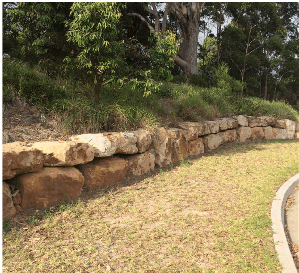
Retaining Wall, Bulli
