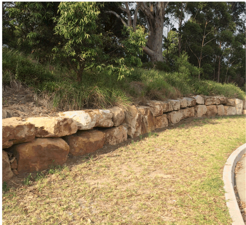
Retaining Wall, Bulli
